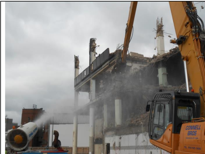
Dust Boss producing a fine mist to suppress dust Town Centre Demolition
