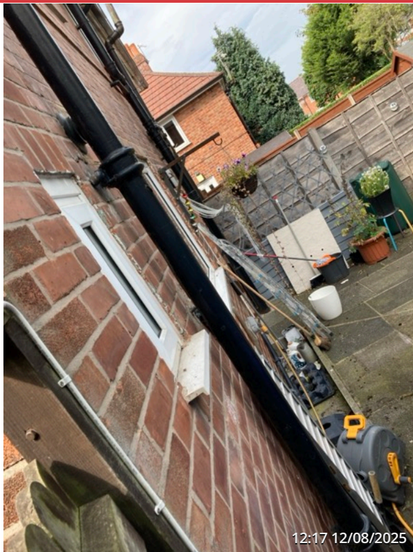
IMAGE 10 Rear of property
