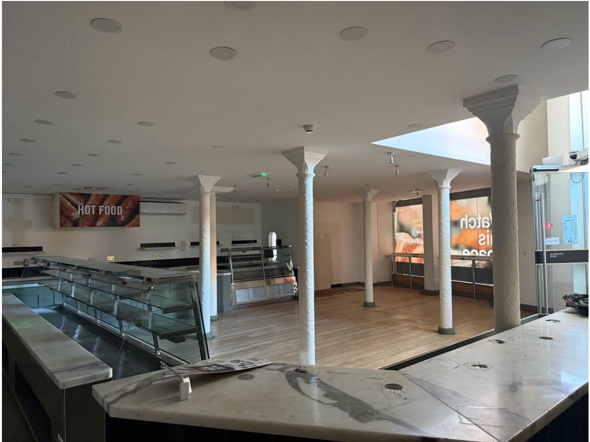
FIGURE 2.10 SITE PHOTOGRAPH OF GROUND FLOOR SHOWING EXISTING FINISHES
