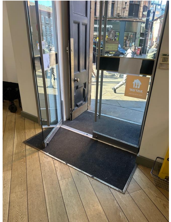
FIGURE 2.7 SITE PHOTOGRAPH OF GROUND FLOOR SHOWING EXISTING ENTRANCE DOORS TO BE RETAINED
