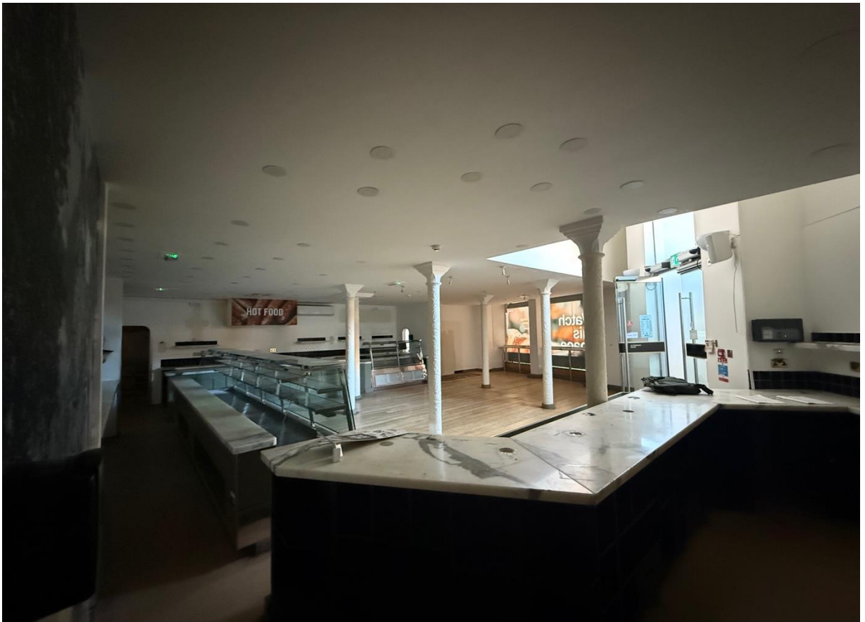
FIGURE 2.8 SITE PHOTOGRAPH OF GROUND FLOOR SHOWING EXISTING CEILING TO BE RETAINED
