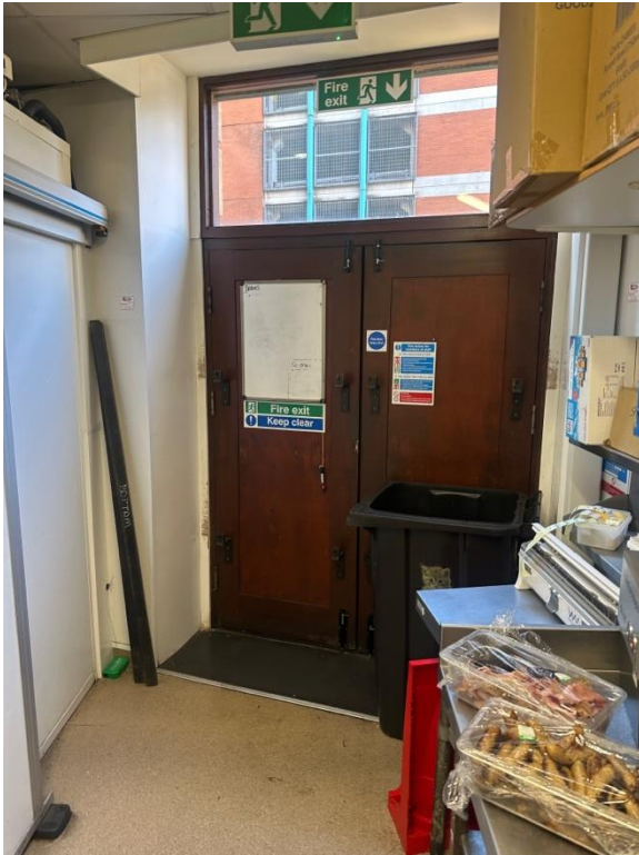
FIGURE 2.6 SITE PHOTOGRAPH OF GROUND FLOOR SHOWING EXISTING DELIVERY DOORS TO BE RETAINED
