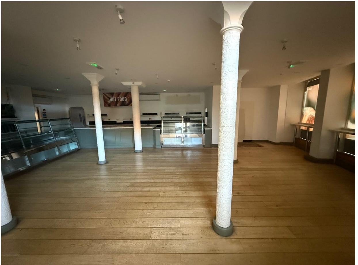
FIGURE 2.9 SITE PHOTOGRAPH OF GROUND FLOOR SHOWING EXISTING FLOOR FINISHES
