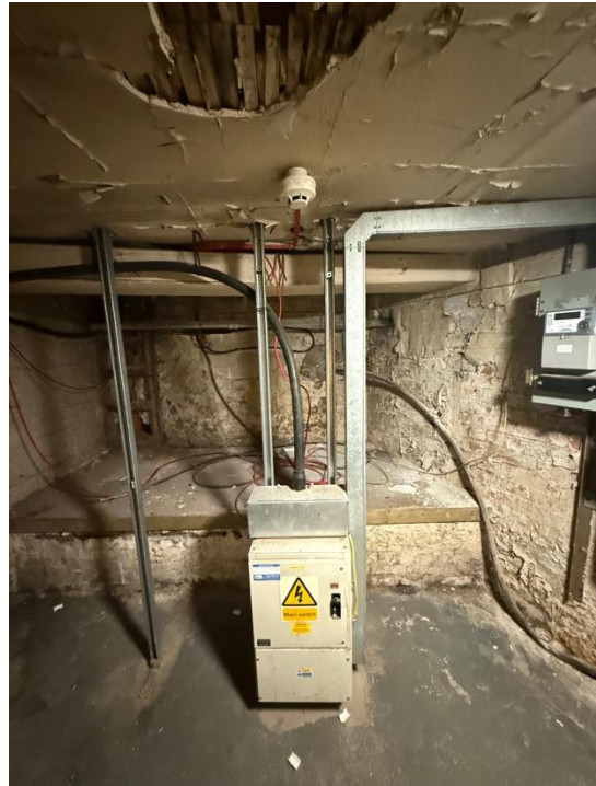
FIGURE 2.4 SITE PHOTOGRAPH OF BASEMENT SHOWING ORIGINAL LATH & PLASTER CEILING
