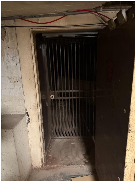
FIGURE 2.1 SITE PHOTOGRAPH WITHIN BASEMENT OF ORIGINAL METAL GATE
