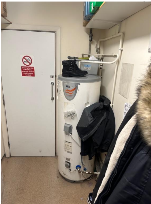
FIGURE 4.18 EXISTING STAFF TOILET AREA TO BE RECONFIGURED FOR NEW CUSTOMER DISABLED TOILET
