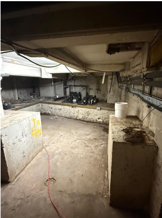
FIGURE 2.11 SITE PHOTOGRAPH OF BASEMENT FLOOR SHOWING EXISTING PLANT
