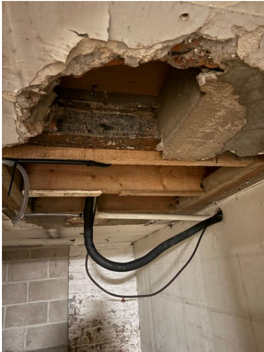
FIGURE 2.3 SITE PHOTOGRAPH SHOWING EXISTING CEILING OPENINGS FORM&E SERVICES
