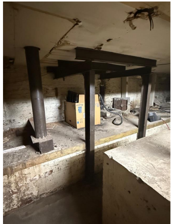
FIGURE 2.2 SITE PHOTOGRAPH WITHIN BASEMENT OF THE REPAIRS TO THE EXISTING STEEL COLUMN
