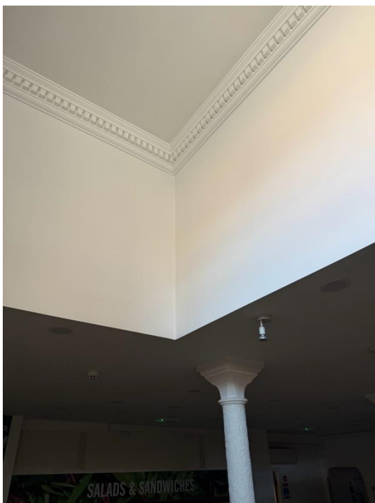
FIGURE 2.5 SITE PHOTOGRAPH OF GROUND FLOOR SHOWING NEW CORNICE INSTALLED BY PREVIOUS OCCUPIER
