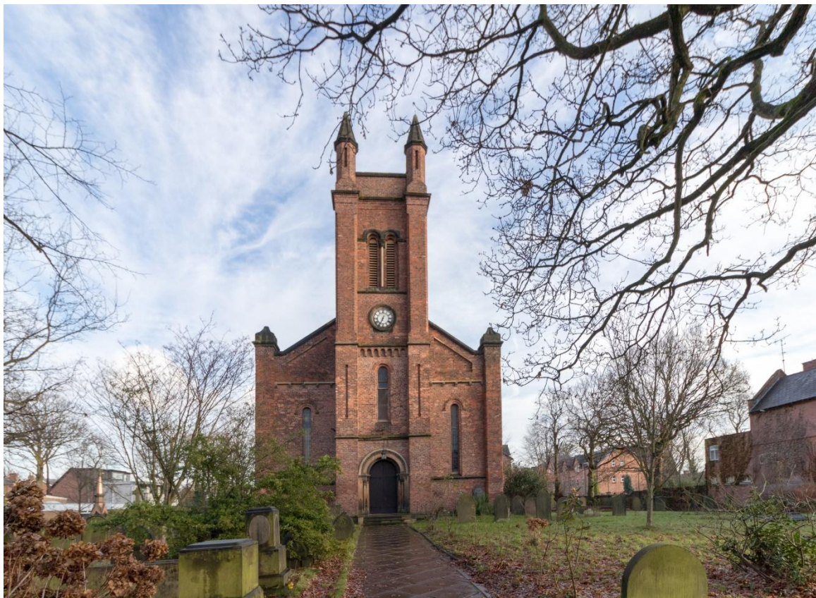
Figure 5-4 Church of St Paul principal façade from Wilmslow Road (Image: Barrie Price, via Historic England List Entry)
