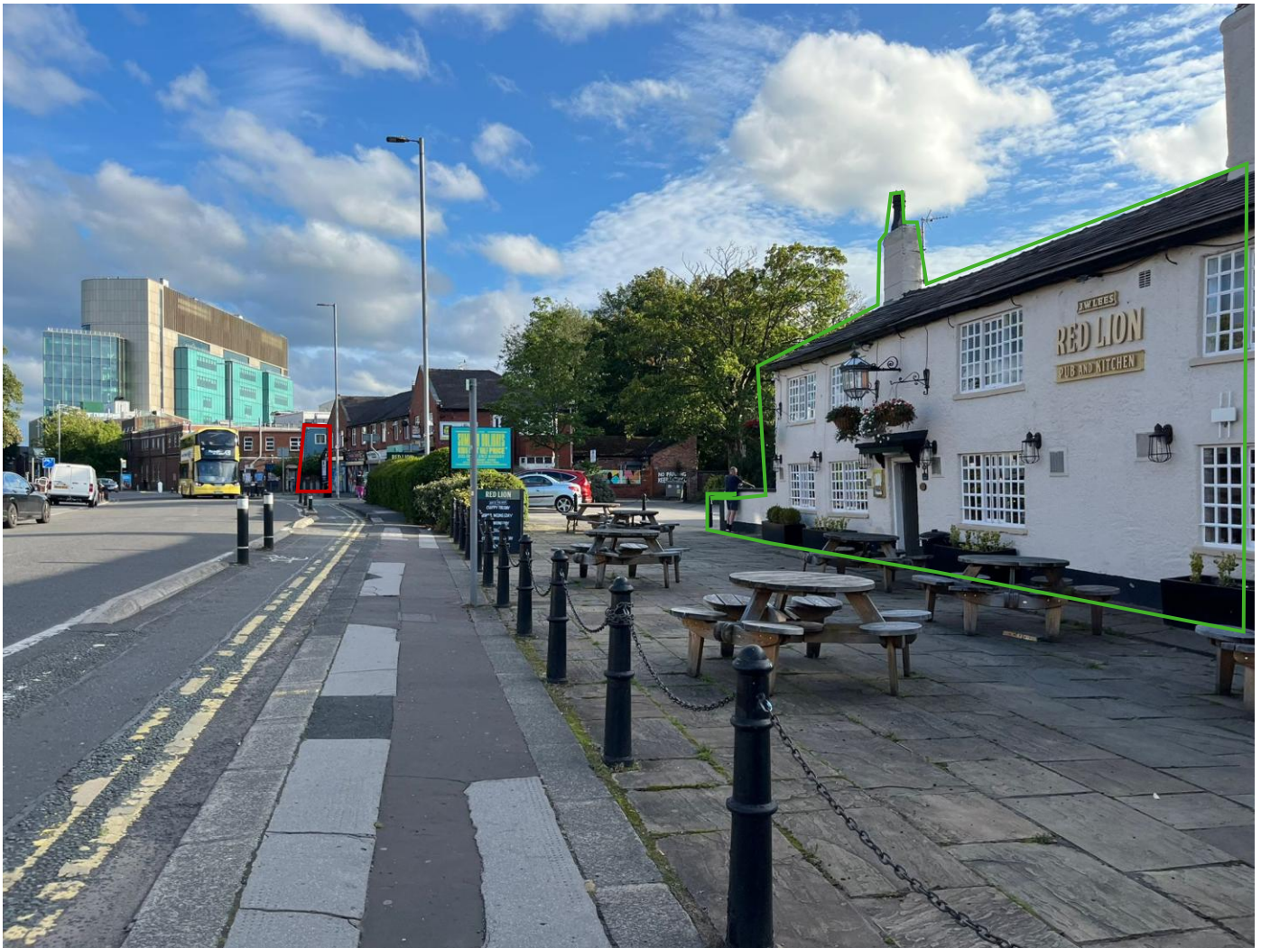
Figure 5-1 Front View of Red Lion Inn, heritage asset (outlined in green) in conjunction with the Site (outlined in red). (Photo taken July 2025, Authors own)
