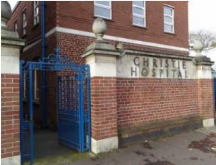
Figure 2-3 Retained frontage including walls and gate.
