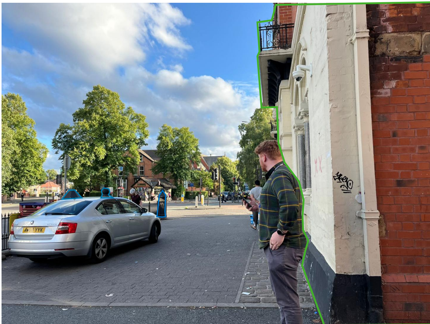
Figure 4-5 View of former White Lion Public House heritage asset (outlined in green), Pairs of Stone Piers heritage assets (outlined in blue). Photo taken looking south towards the Site. (Photo taken July 2025, Authors own)
