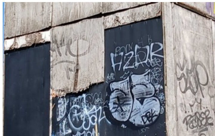
Image 8: Lifted wooden panelling along the maintenance unit
