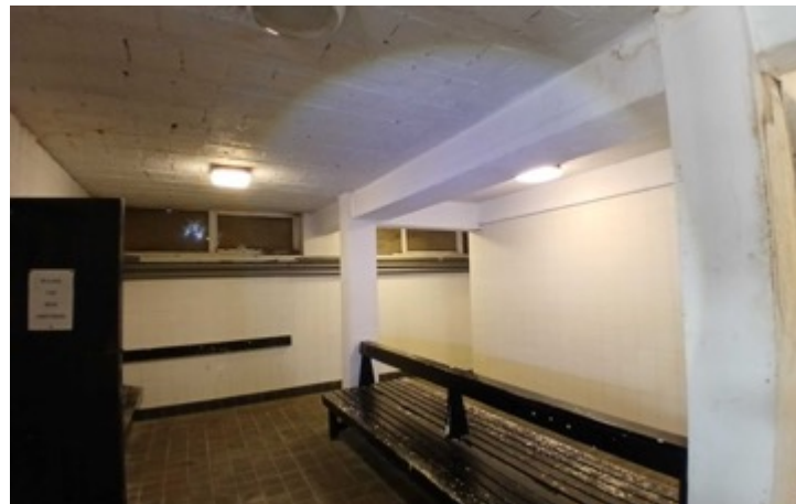
Image 6: Internal space of B1
