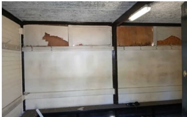
Image 5: Internal space of B1
