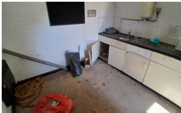
Image 7: Internal space of B1
