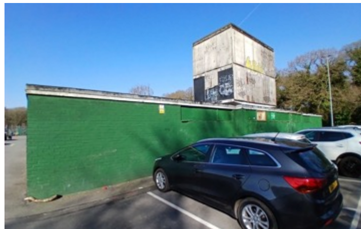
Image 2: Eastern elevation of B1
