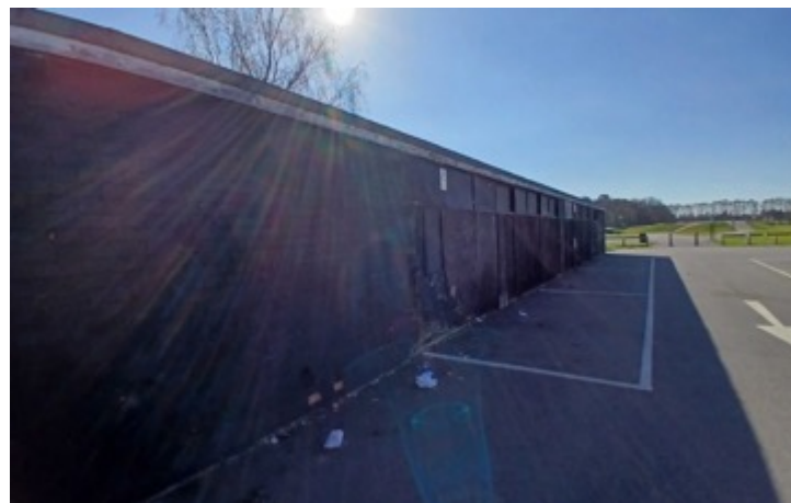
Image 4: Western elevation of B1
