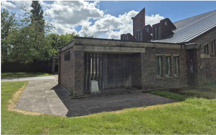
Original Main Entrance View from North-East
