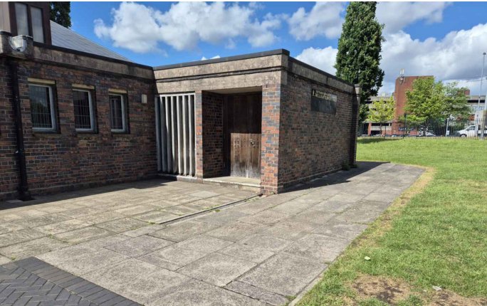
Original Main Entrance View from South
