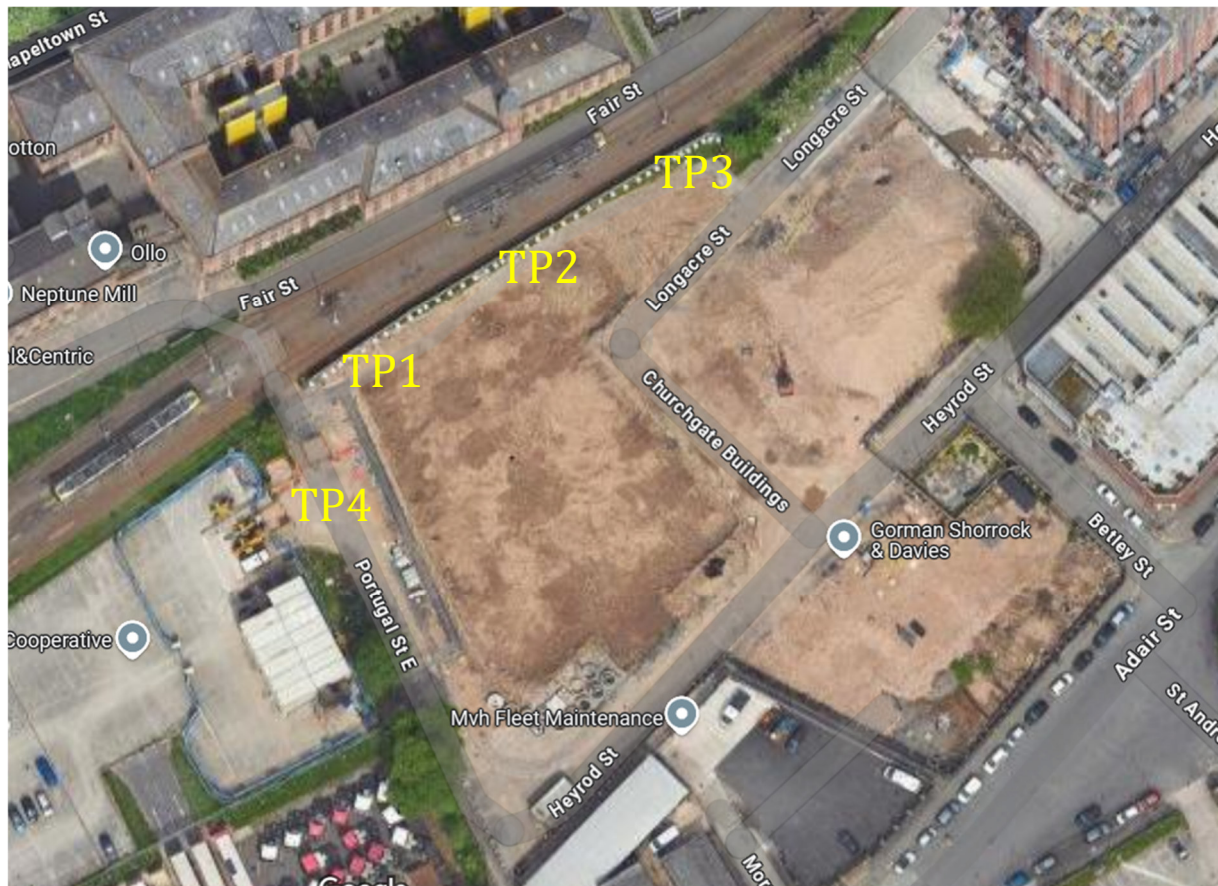
Figure 1. Site of Fairfax buildings (shown prior to any construction work).
