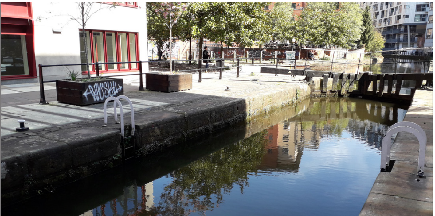
View of the timber lock gates and sandstone edging to the canal
