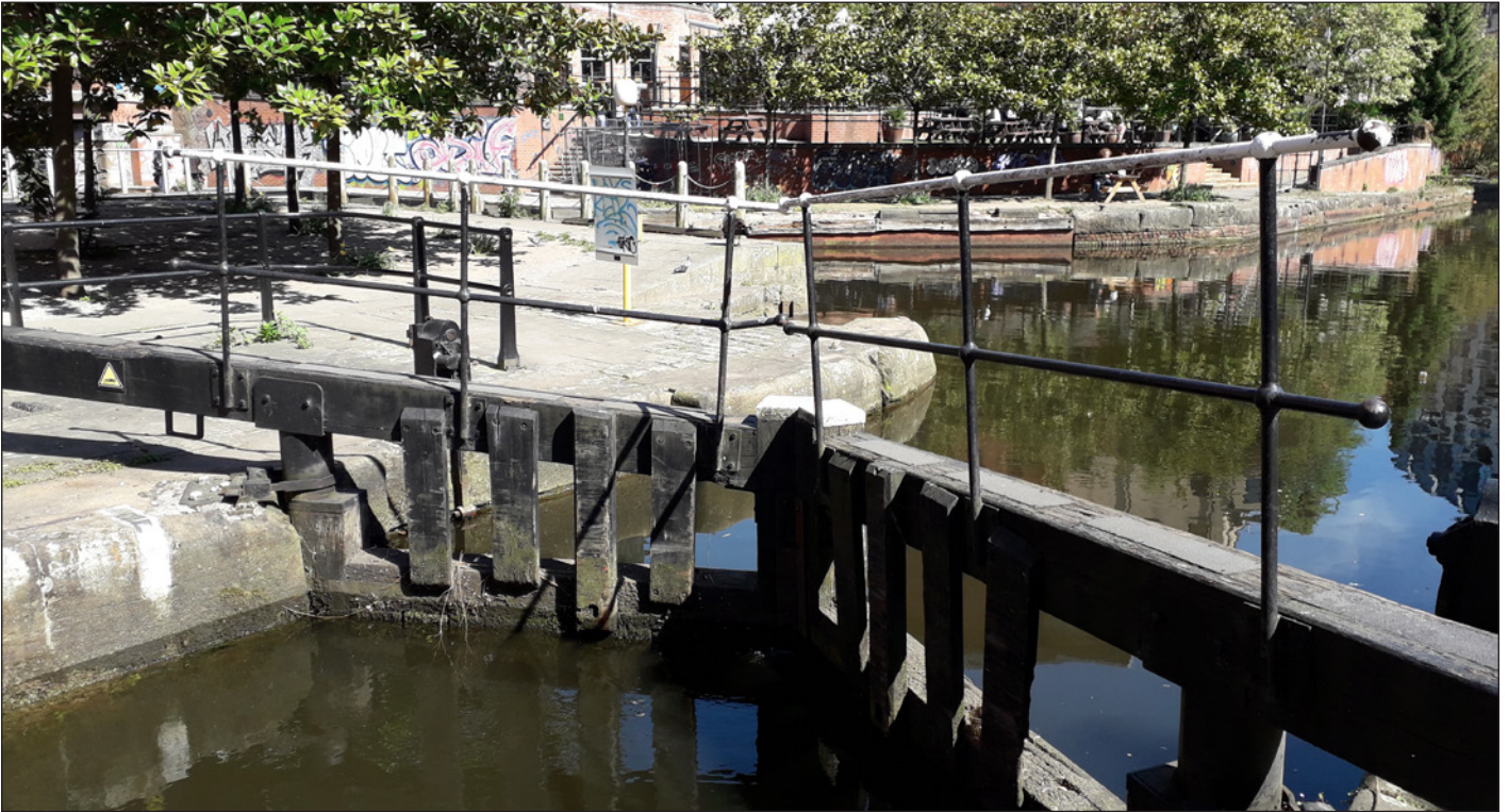
View of Lock 89 (Tib Lock) gate and proposed area for new guardrail (as viewed towards the north east)
