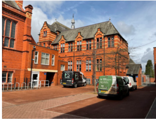
3.17 1886 building (R), south elevation, to the courtyard
