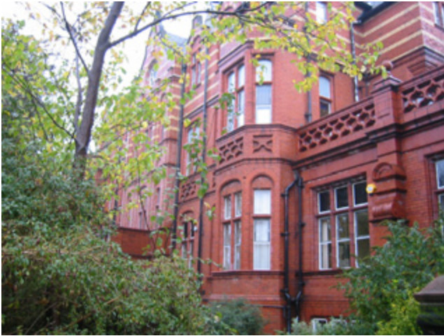
3.16 1886 building, detail of the west elevation
