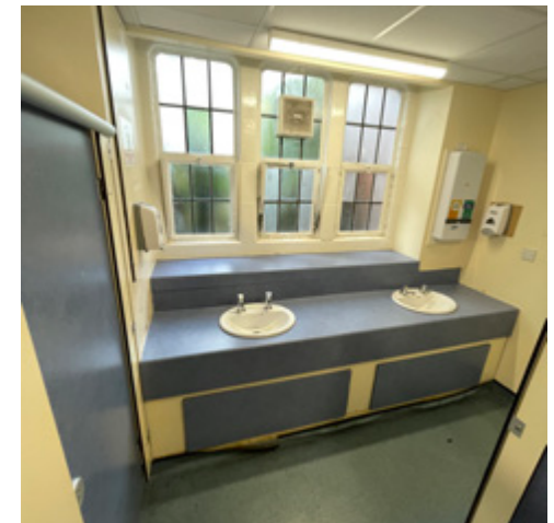
3.34 1886 building Basement, Girls' WCs (CoARC)
