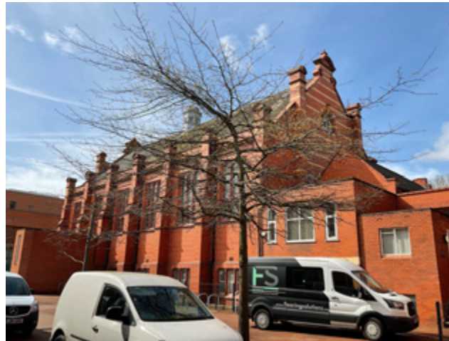
3.19 1910 building, east (rear) elevation
