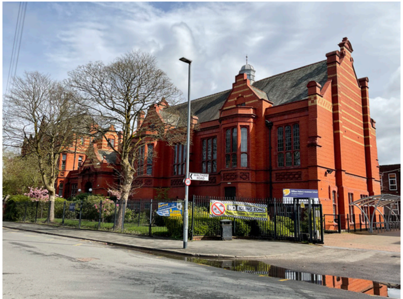
3.1 1886 (L) and 1910 (R) buildings, west (principal) elevation, to Spring Bridge Road
