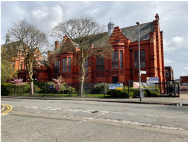
3.18 1910 building, west (principal) elevation, to Spring Bridge Road
