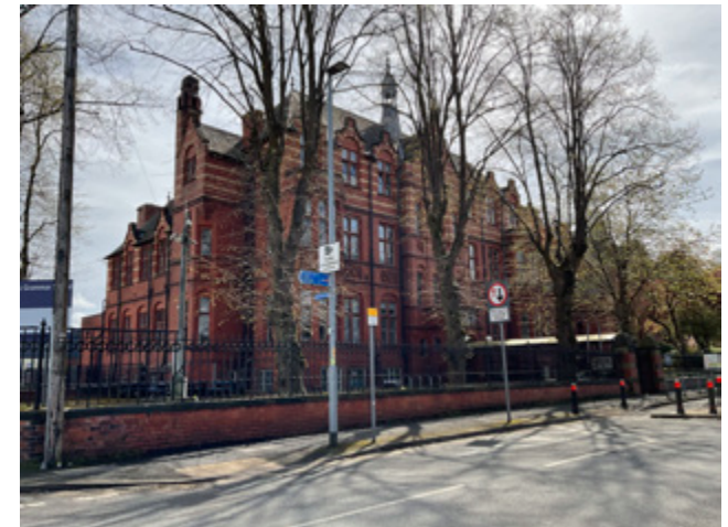
3.15 1886 building, north (L) and west (principal, R) elevations
