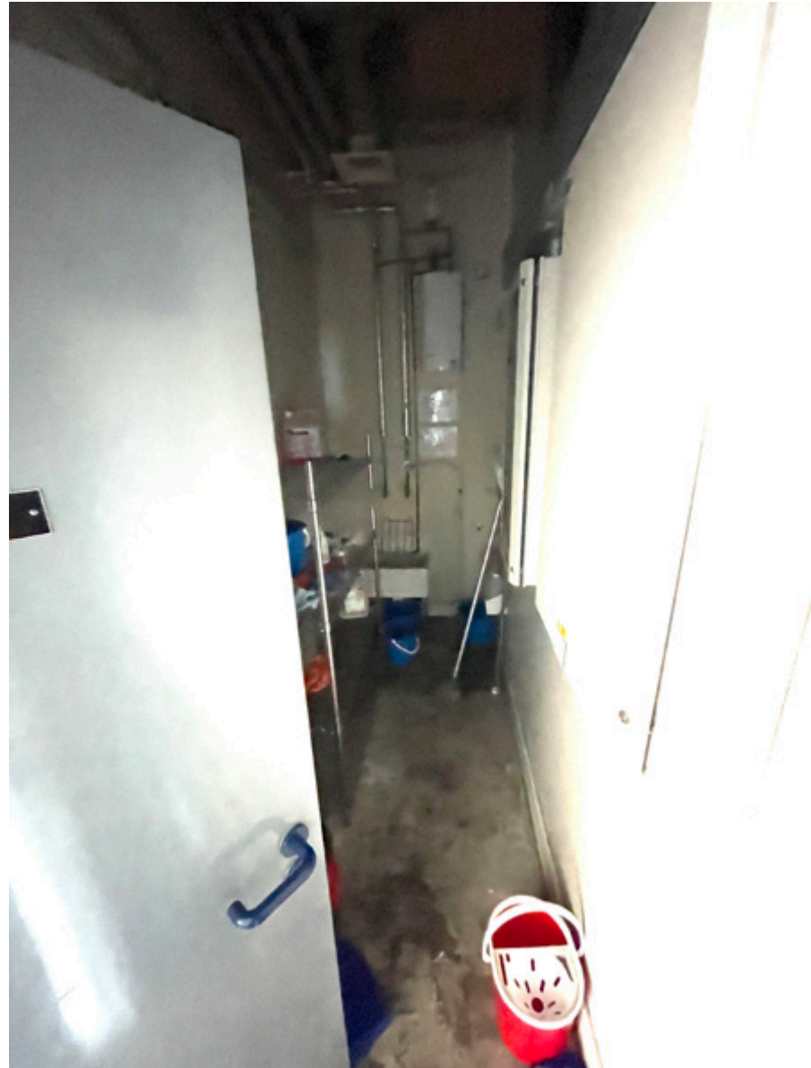
3.44 Science Building, Cleaner's Store (CoARC)
