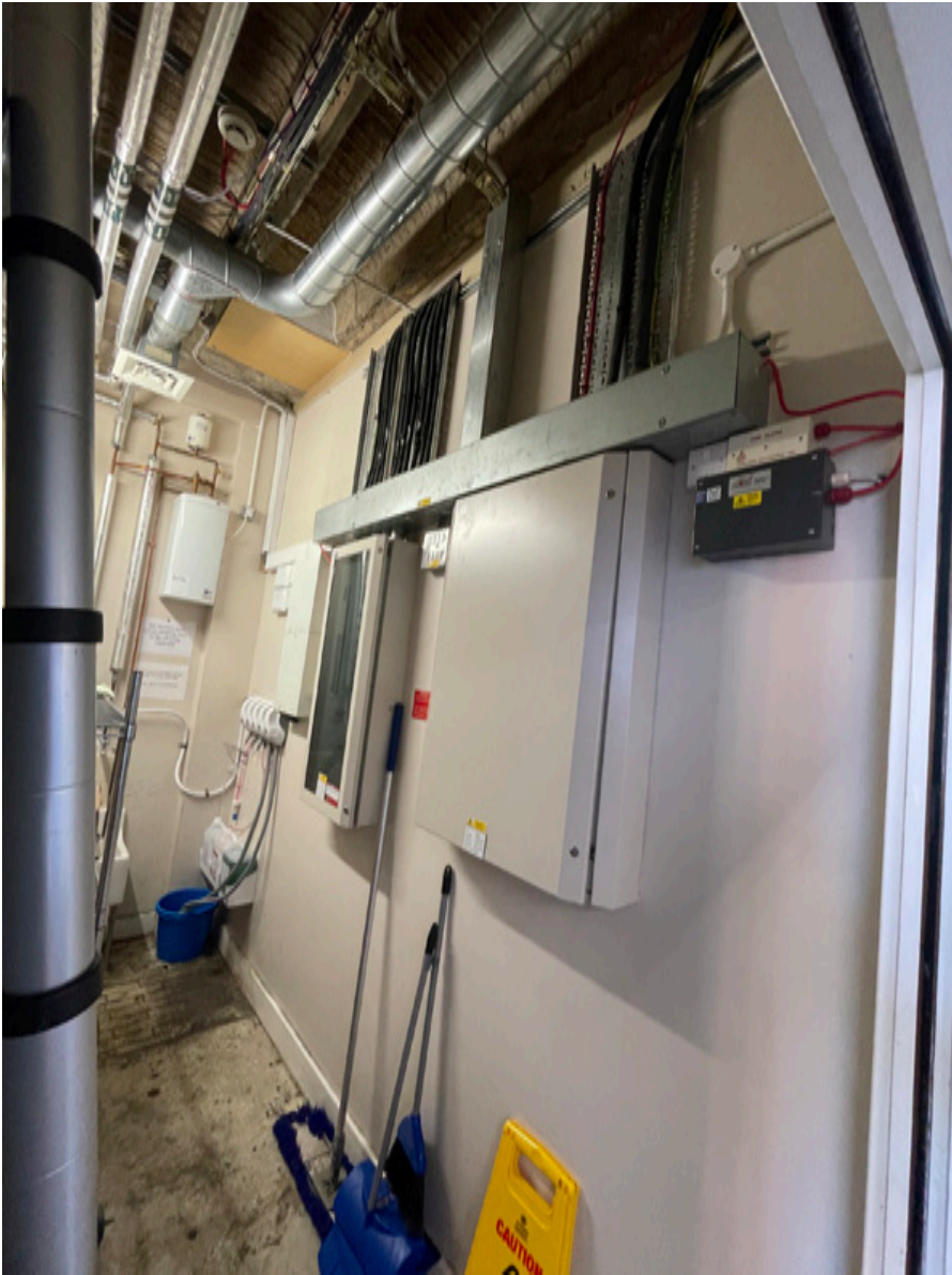
3.43 Science Building, Cleaner's Store (CoARC)
