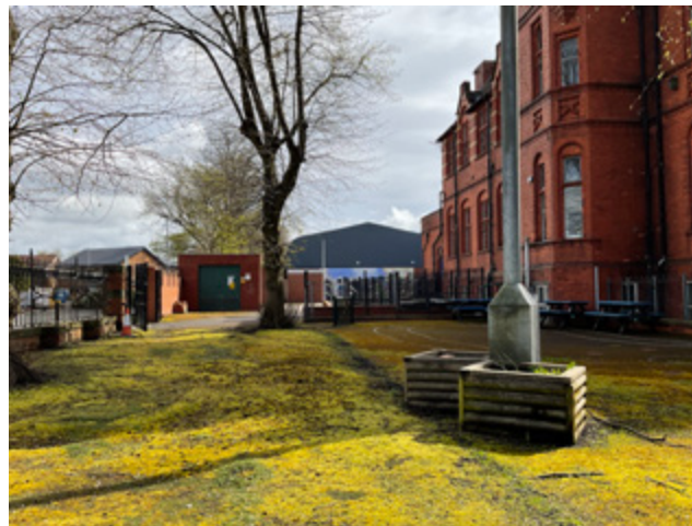
3.12 Substation and Sports Hall visible to the rear of the north frontage
