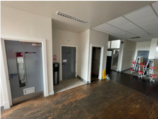
3.38 Science Building, entrance area (CoARC)
