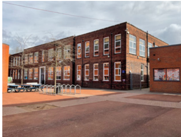
3.35 Science Building, west elevation, to the Quad
