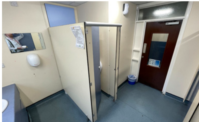
3.33 1886 building Basement, Girls' WCs (CoARC)
