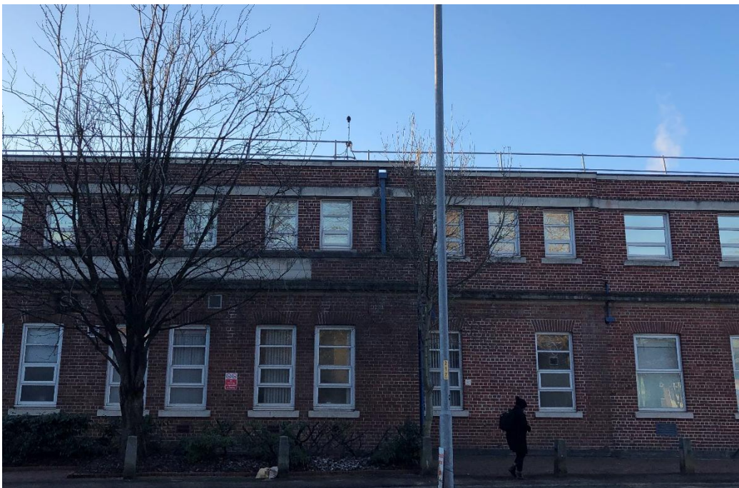
Figure 4 Unattended measurement equipment - seen from Wilmslow Road
