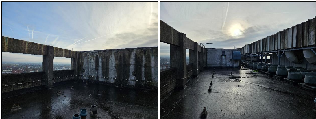
Photographs 8 (left) and 9 (right) showing the roof.
