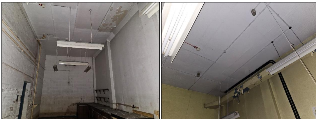
Photographs 3 (left) and 4 (right) showing the interior of the basement floor.
