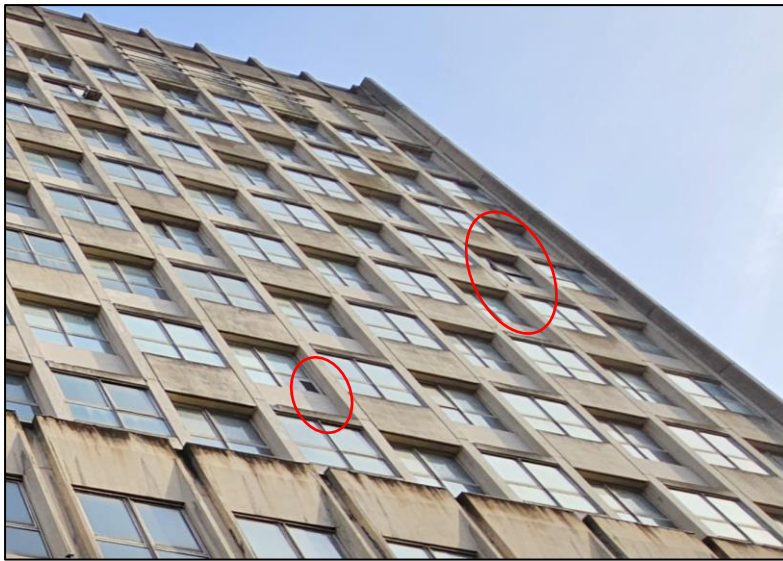
Photographs 1 showing external access points on western elevation.
