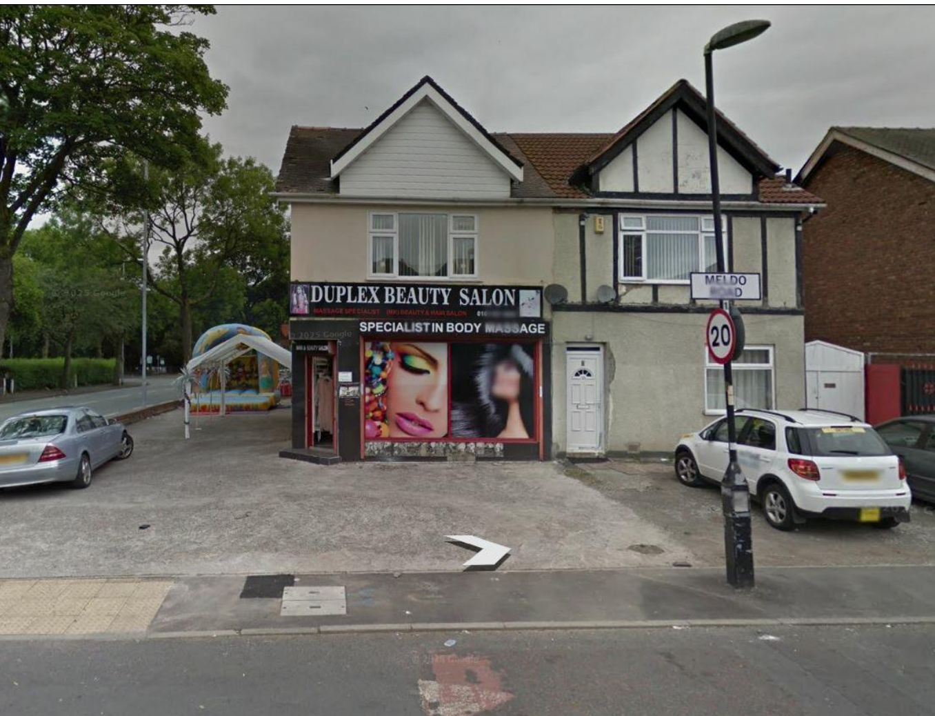
Existing front car park space
