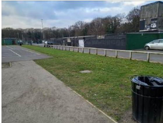
Photo 1— Disused building in centre of existing car park
