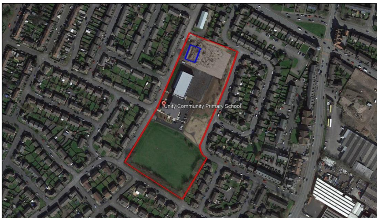
Figure 2-C: Aerial imagery dated 2017 showing stockpiling of soils in the PlayZone area (blue)
