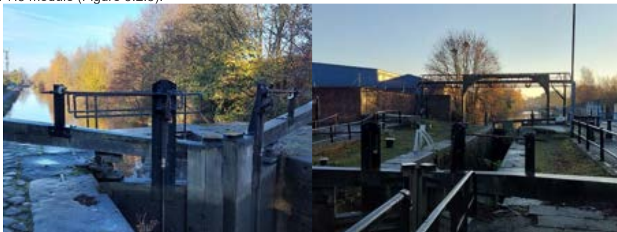
Figure 3.2.3 Canal locks within the MoRPH5
