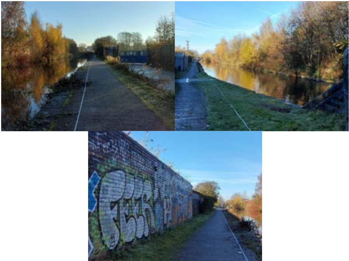
Figure 3.2.1 Photographs of the left bank
