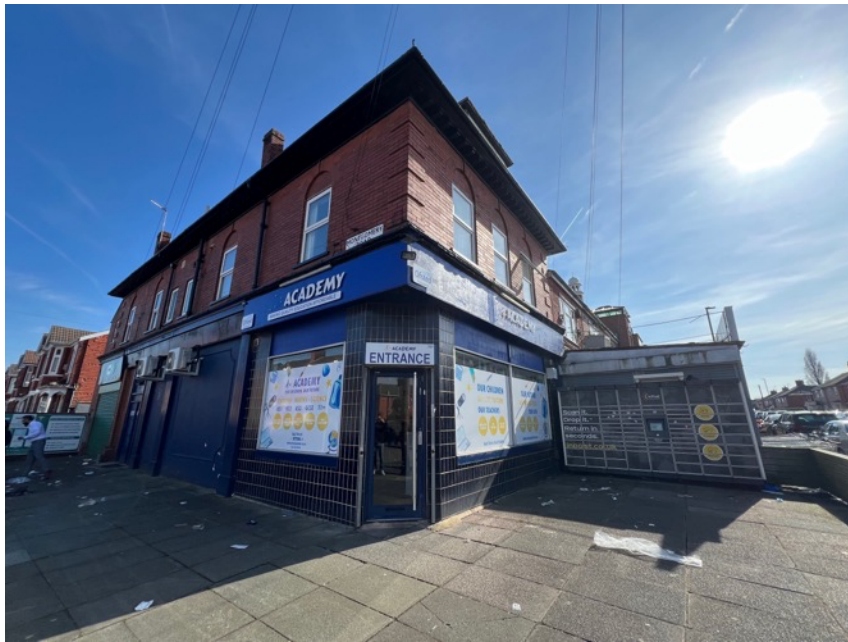
Front of the existing building viewed from the corner of Beresford Road and Montgomery Road.
