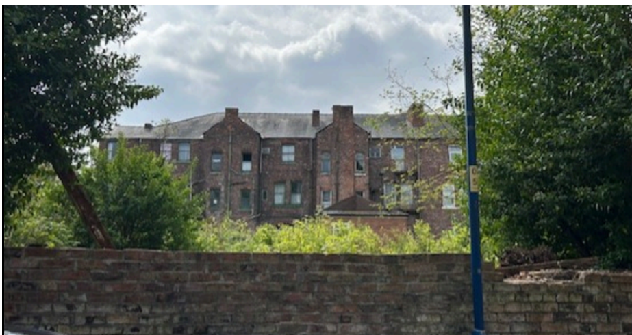
View of application property rear
