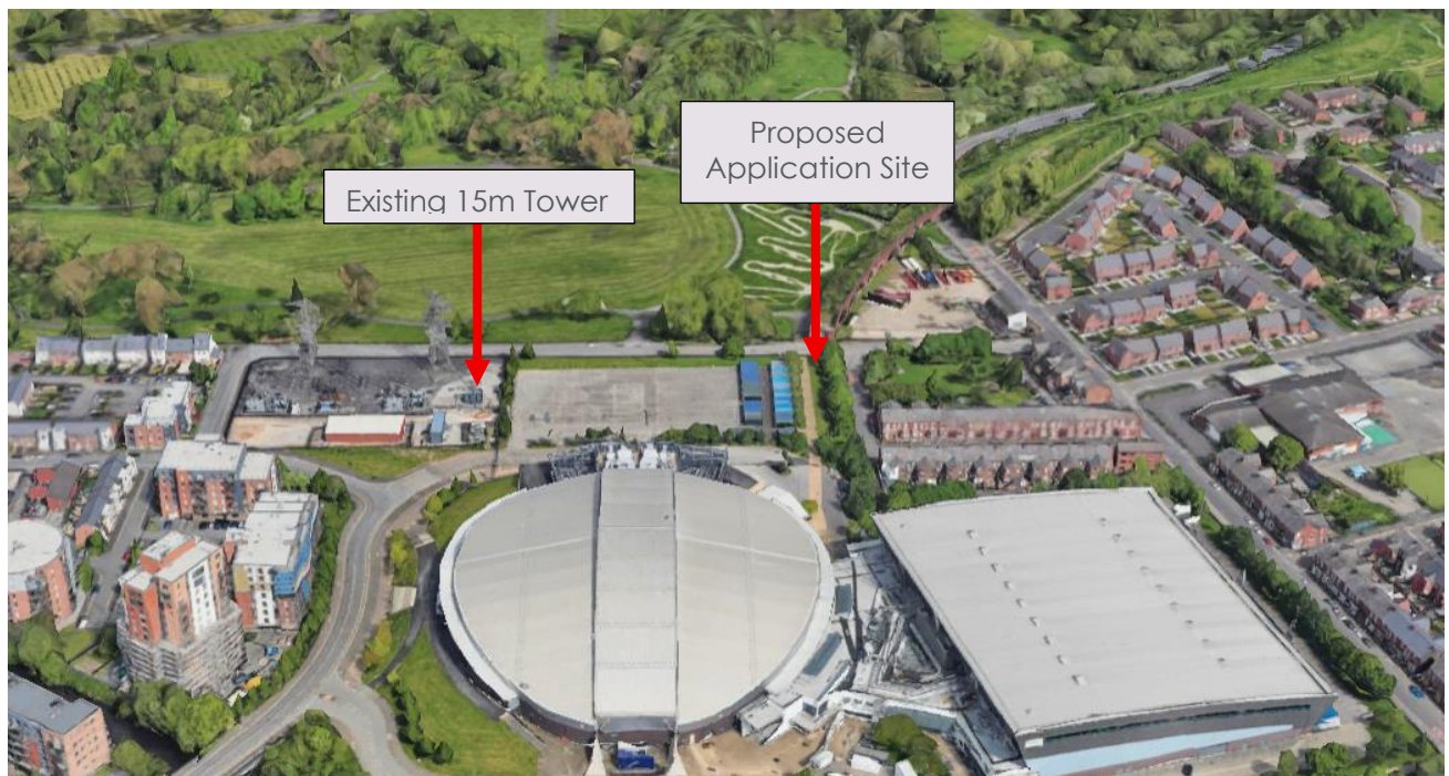
(Figure 2: Aerial View of application site in relation to the existing installation)
