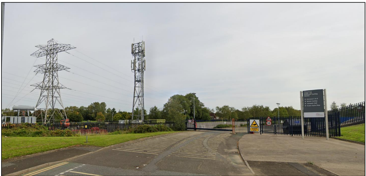
(Figure 1: Street view of the existing shared installation)
