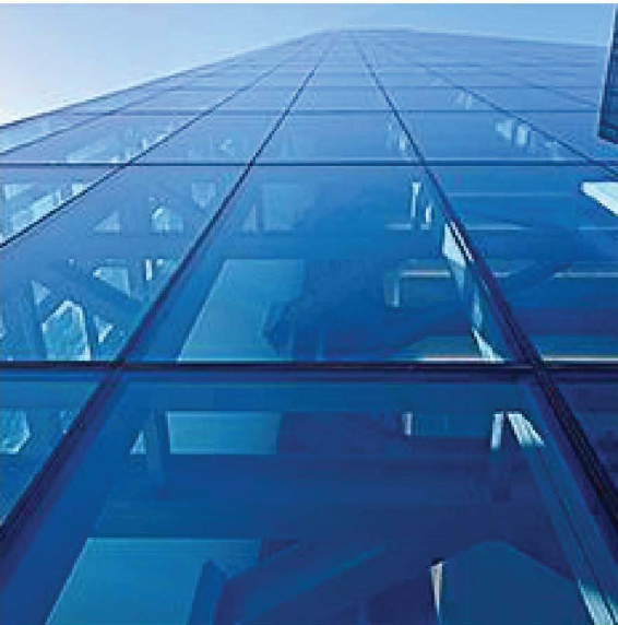
5. Curtain wall glazing
