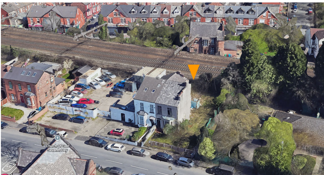
Fig. 1 Aerial view of site.
