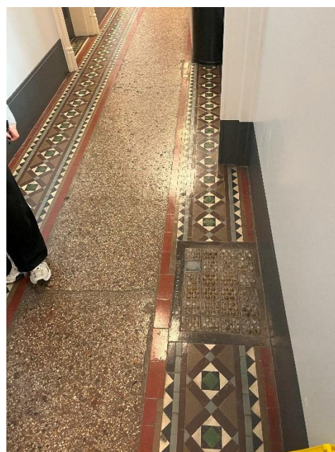
Fig 2.4 Patterned encaustic tiles and terrazzo flooring to the corridor.
