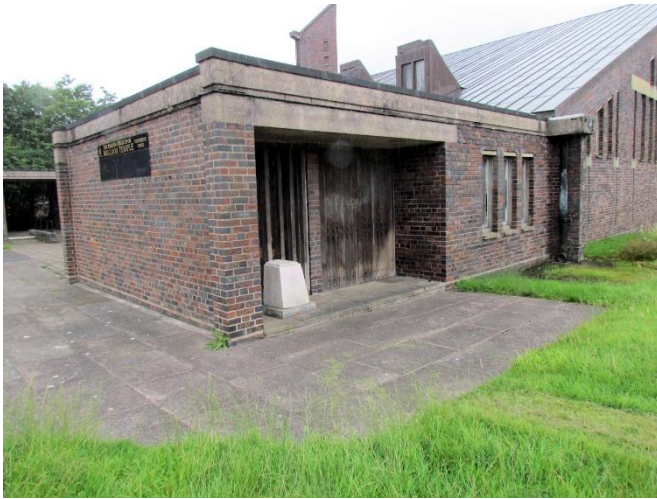
Existing Concrete Paving Around Porch
