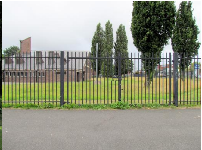
Gates in Perimeter Fence on North-west Side
