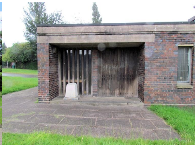
South-east Porch with External Door
