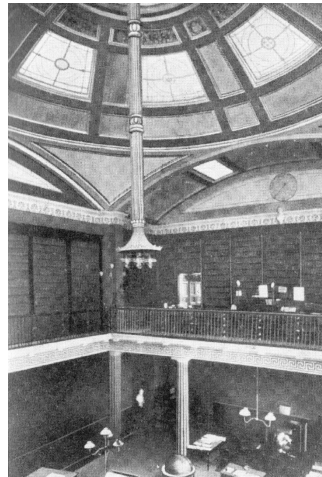
Interior before the 1920s alterations, showing the gasolier of c.1875. The floor aperture was subsequently infilled to accommodate the bank to the ground floor.
