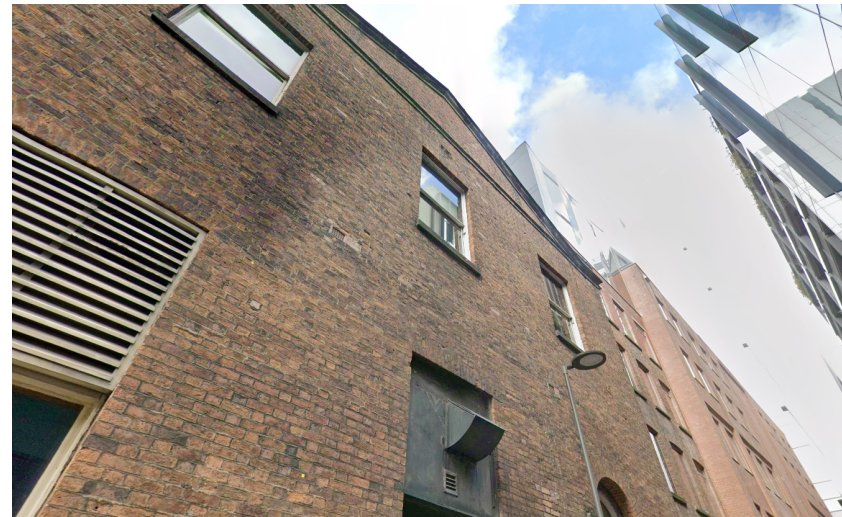
View 04 Narrow Character of Back George Street prevents views of ASHP enclosure. Note extent of extract vents, removal will enhance setting on Back George Street.
