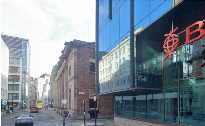
View 01 Looking north-west along Charlotte Street. Rear elevation concealed by the Bank of China.
