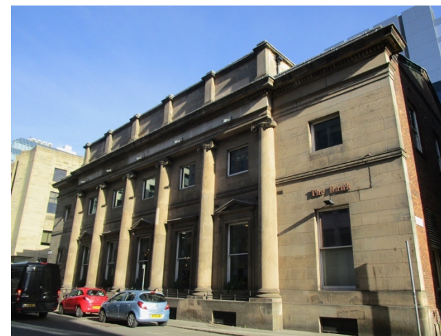
General view of the Portico from Charlotte Street, the first floor windows were inserted into formerly blank panels c. 1920. The ground floor windows had lost their original glazing bars by the late C19.
