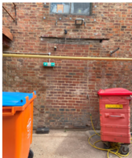
Existing bricked up fire escape door
