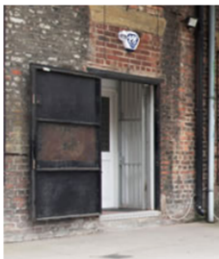
Main entrance door
