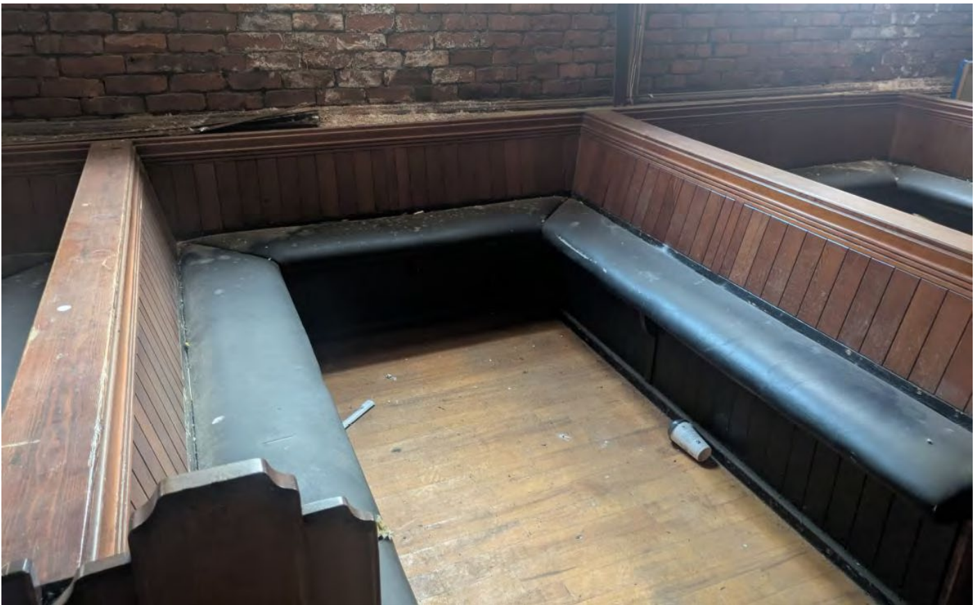
The Historic Pews and Joinery
