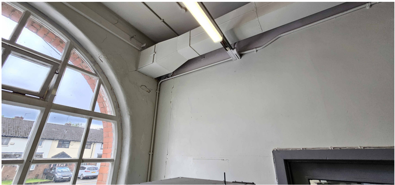
Image 2 - Existing wall penetration
