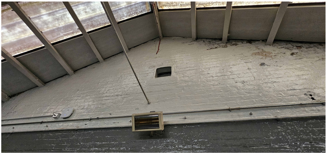
Image 3 - Existing wall penetration
