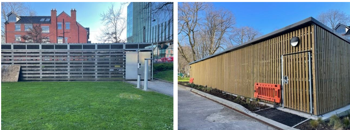
Figure 3-9 – Nearby Cycle Parking Hubs
