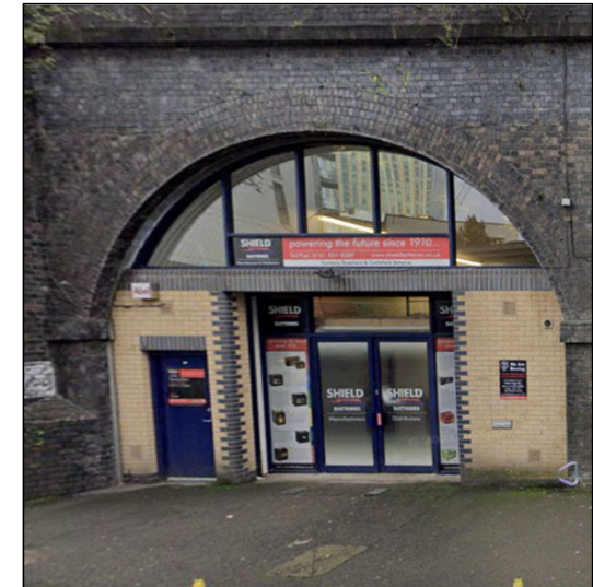
Viaduct Street, Salford
