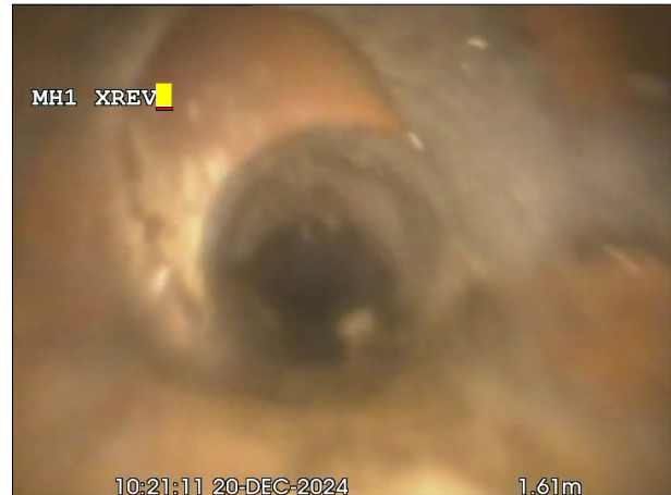
Photo: 2_4a, 00:00:00 1.6m, Junction at 11 o'clock, dia 100 mm
