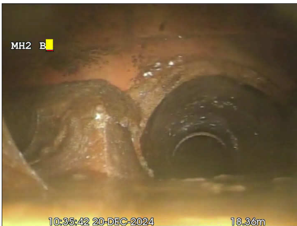
Photo: 5_32a, 00:00:00 18.35m, Finish Survey, Remark: Man Hole Reached
