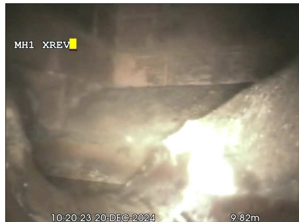
Photo: 13_6a, 00:00:00 9.8m, Finish Survey, Remark: Survey Finished, Man Hole reached
