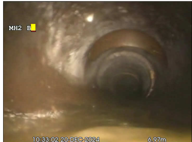
Photo: 5_14a, 00:00:00 7.1m, Junction at 12 o'clock, dia 150 mm
