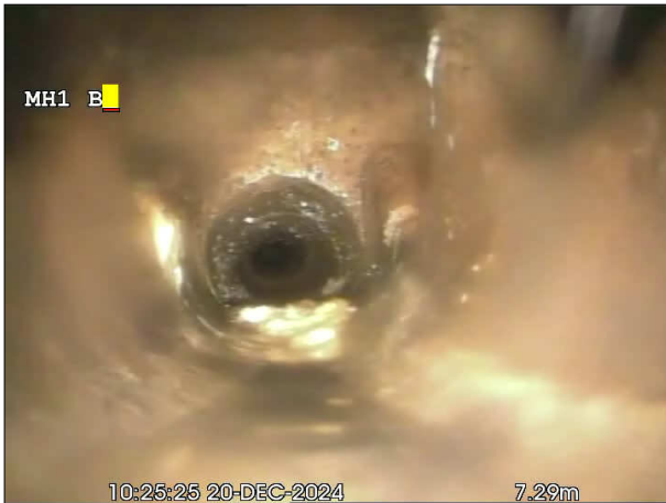
Photo: 4_8a, 00:00:00 7.3m, Finish Survey, Remark: Man Hole Reached
