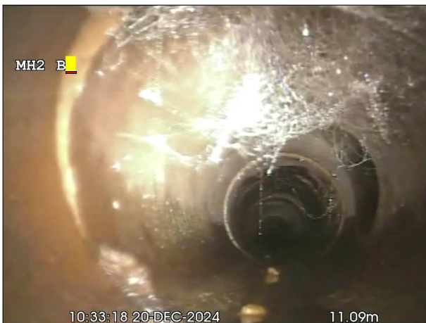
Photo: 5_19a, 00:00:00 11.2m, Junction at 03 o'clock, dia 150 mm
