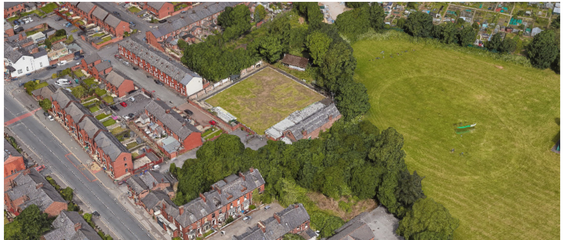
Aerial photographs of application site and context
