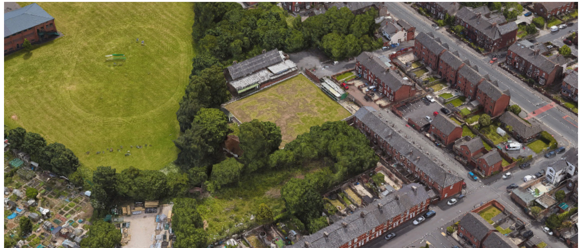
Aerial photographs of application site and context
