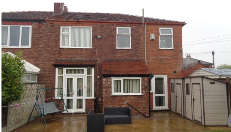
Rear Elevation of Application Property.
