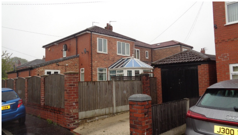
Rear Elevations of Adjacent Property.
