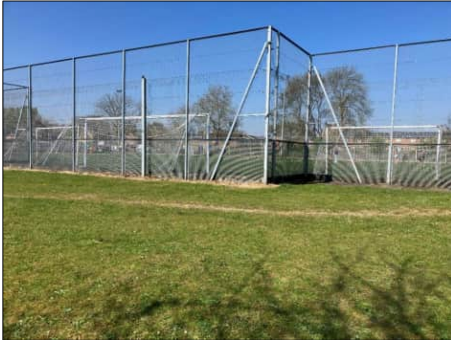
Photograph 5 - Photograph of AGP extension area facing west
