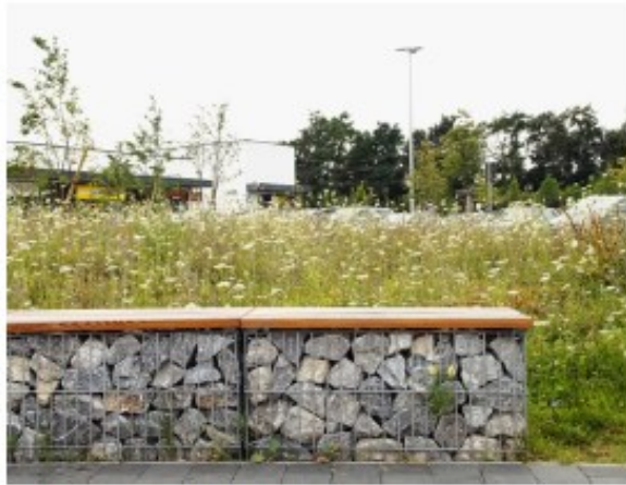
Gabion retaining walls / seat
