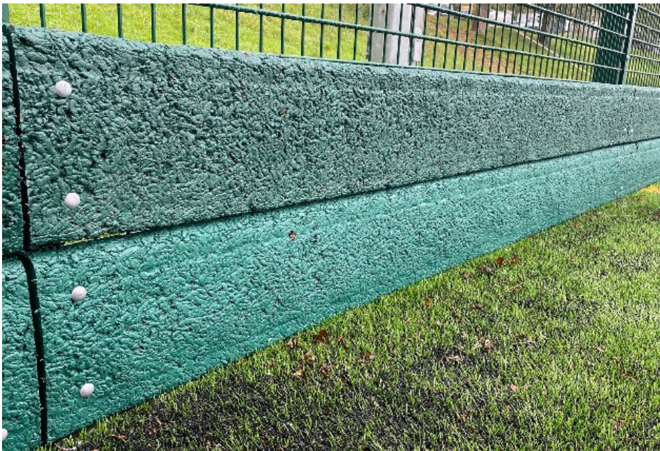
FIGURE 22 Example photographs showing Trekboards which help prevent the spread of rubber crumb. Image credit: SAPCA & NBS
