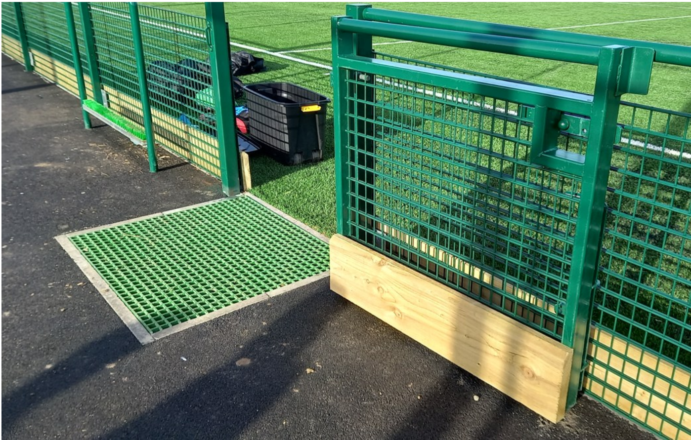
FIGURE 21 Example photograph showing a detox grid (located at pitch entrances)
