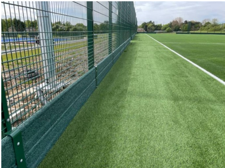
FIGURE 22 Example photographs showing Trekboards which help prevent the spread of rubber crumb. Image credit: SAPCA & NBS
