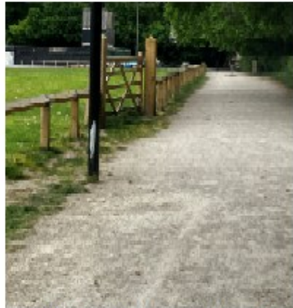
Compacted loose gravel paths to tie in with existing
