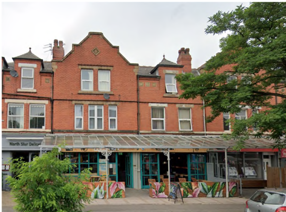
Wilbraham Road frontage of application property dated July 2019
