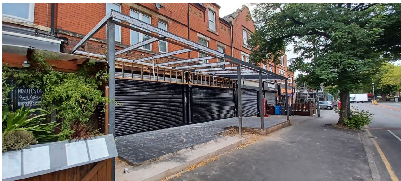
Application site with part-built canopy dated August 2025
