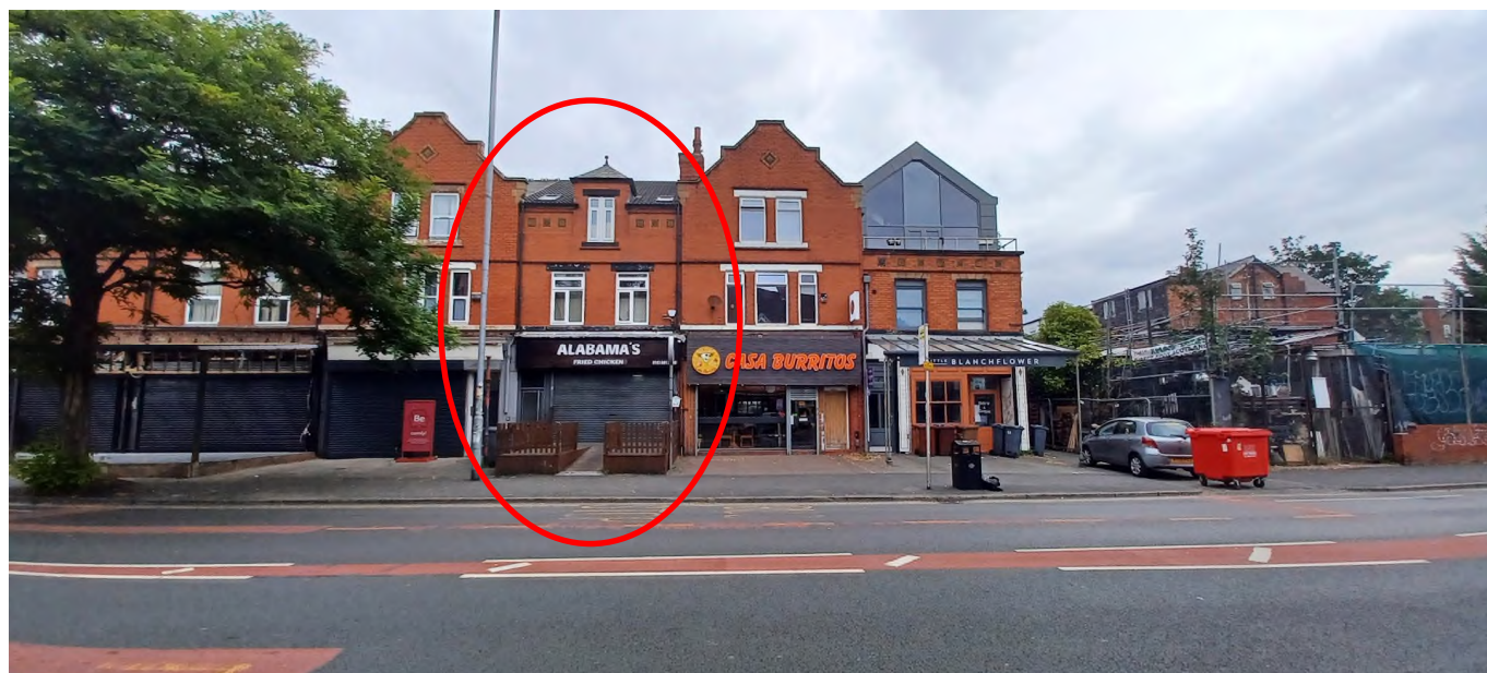
Raised platform at No.410 Wilbraham Road, August 2025
