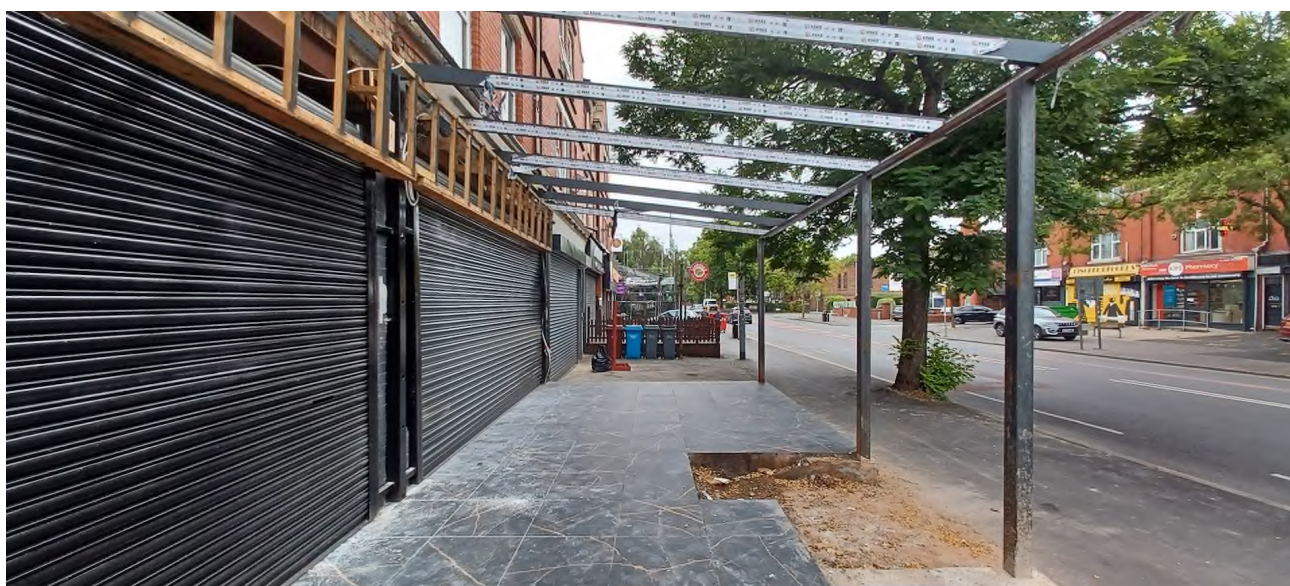
Application site with part-built canopy dated August 2025
