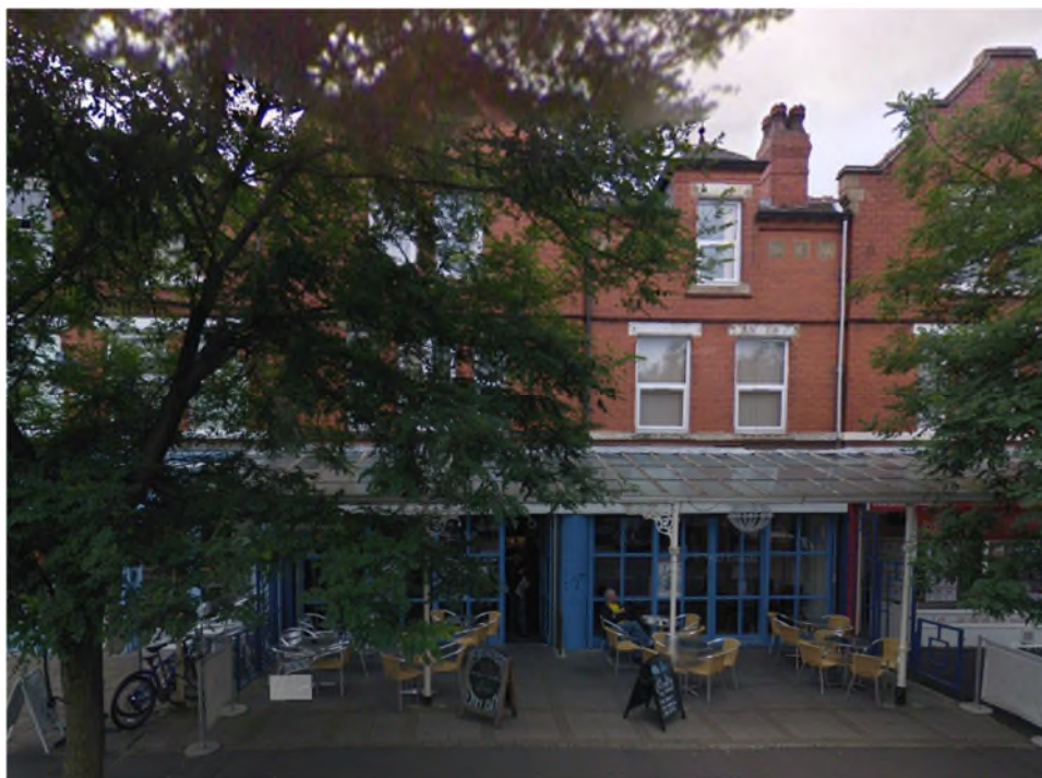
Wilbraham Road frontage of application property dated September 2008
