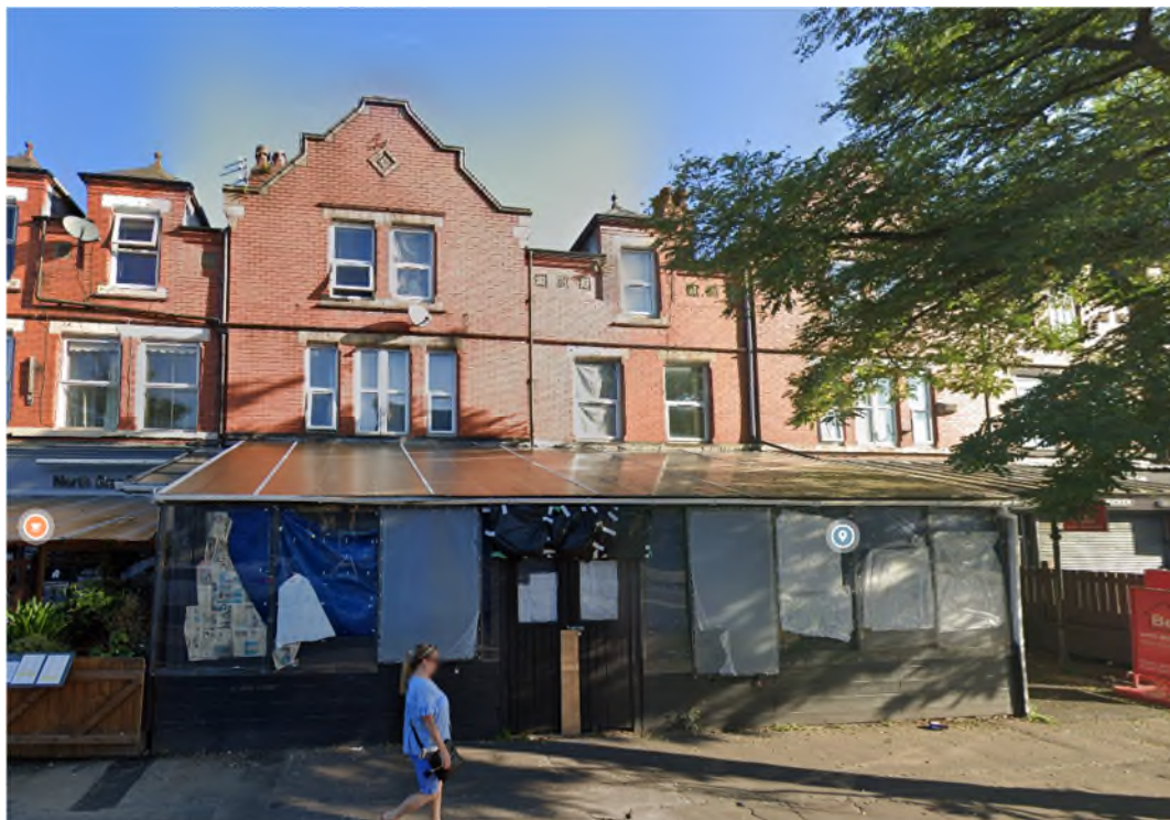
Wilbraham Road frontage of application property dated September 2023
