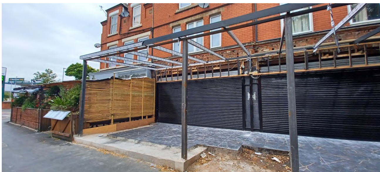
Application site with part-built canopy dated August 2025
