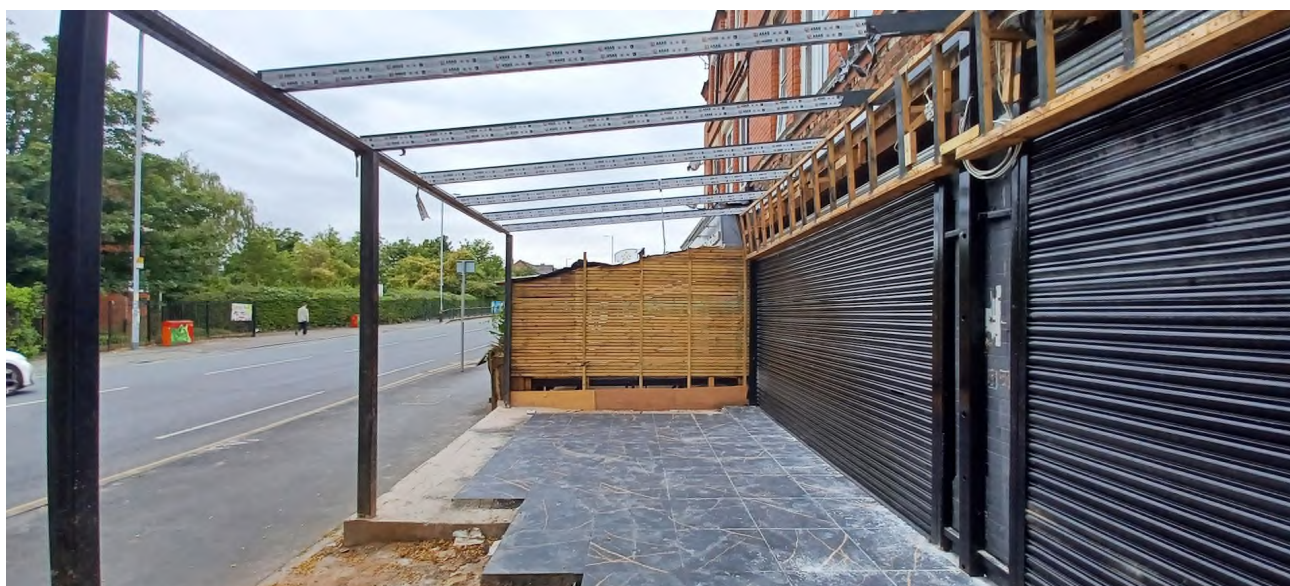
Application site with part-built canopy dated August 2025
