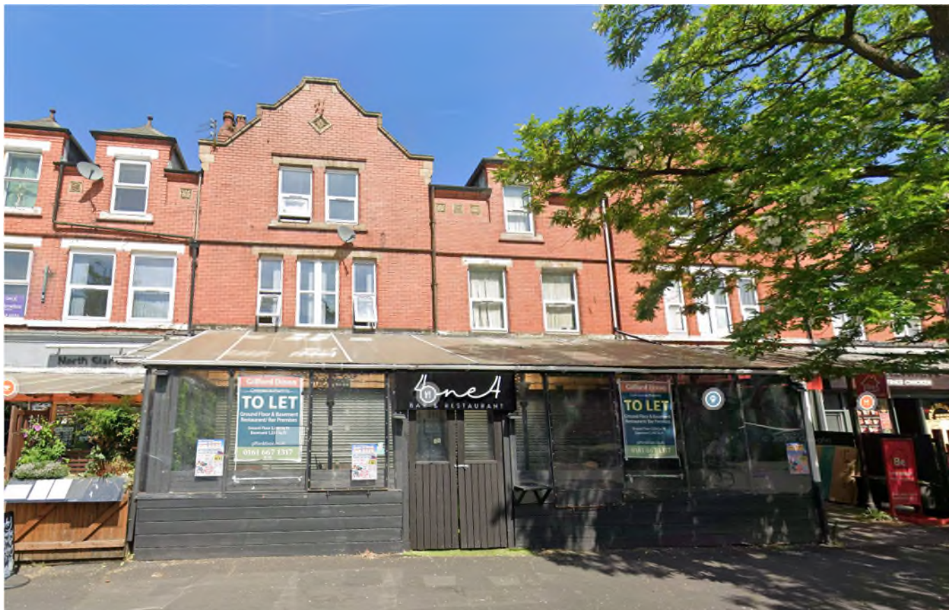
Previous unauthorised canopy present on site dated to May 2025
