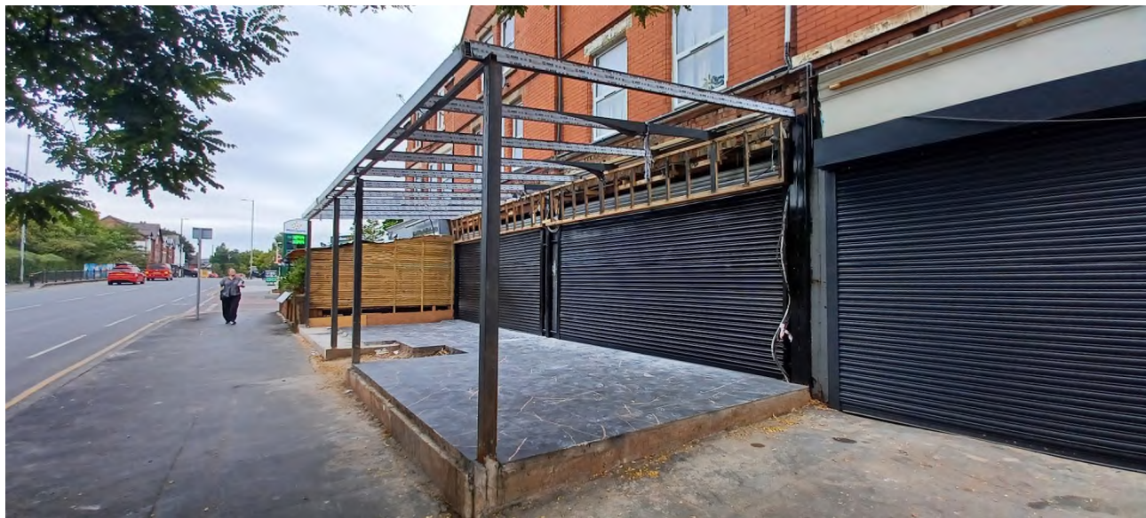
Application site with part-built canopy dated August 2025
