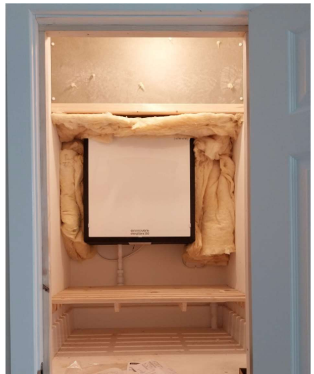
Figure 2-1: Plot 1 Mitigation measures
