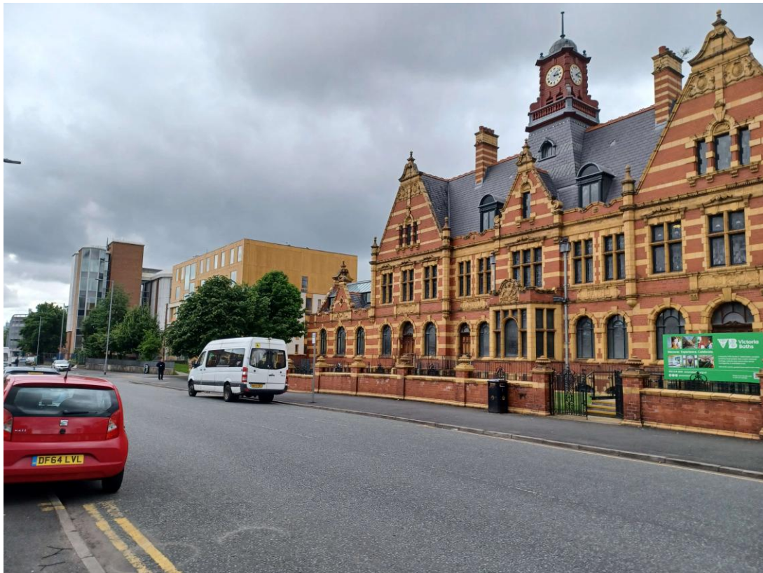
Hathersage Road view of front of site with Octagon House – far left, Block 6 on the application site and Victoria Baths to the right
