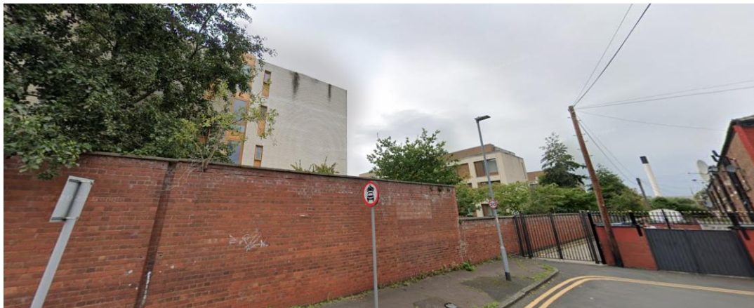
View westwards from Chelford Close /South Grove junction the rear of properties on Upper West Grove to the right and the rears of Blocks 2 and 3 to the left and centre
