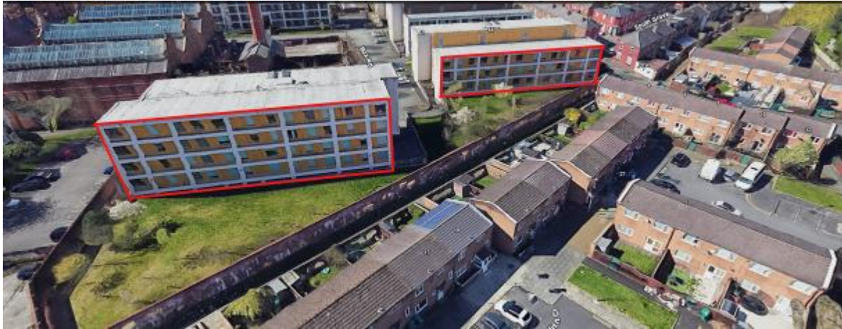
Aerial view towards existing Block 1 (left) and Block 2 (right) and windows on elevations facing towards two storey residential properties on Edbrook Walk
