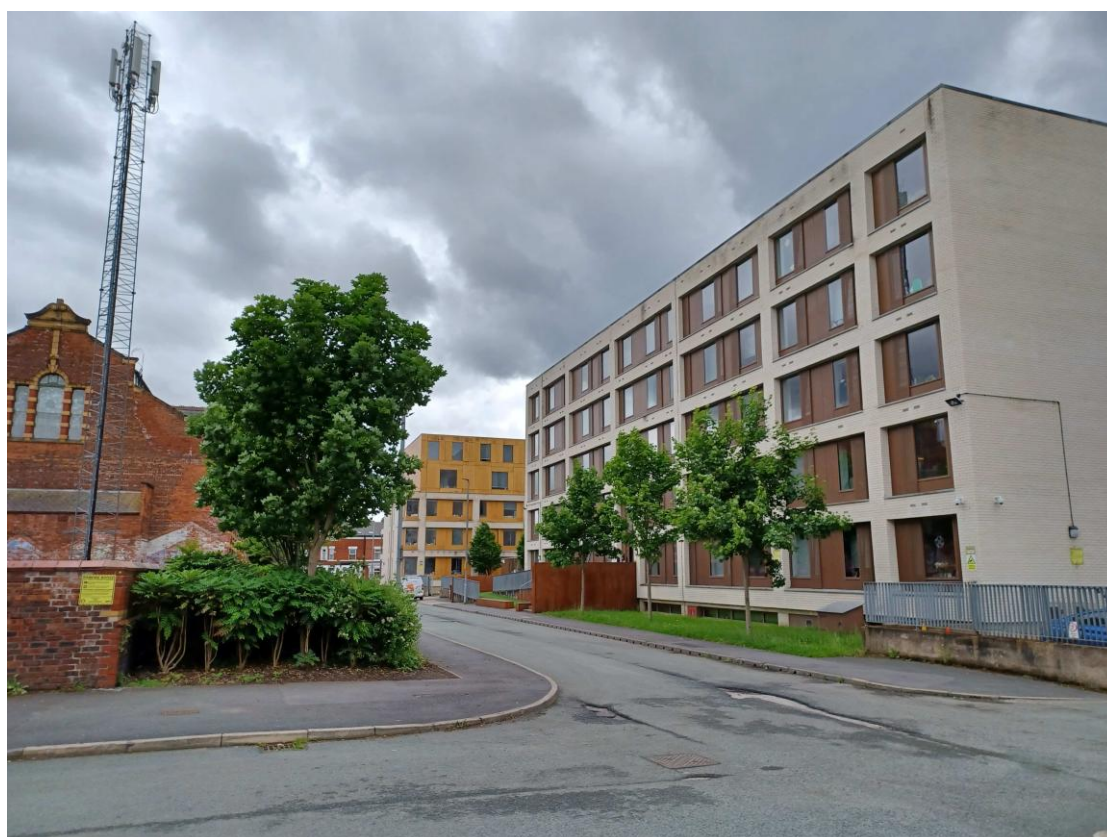
View south along Bax Road with Block 5 to the right and rear of Block 6 centre
