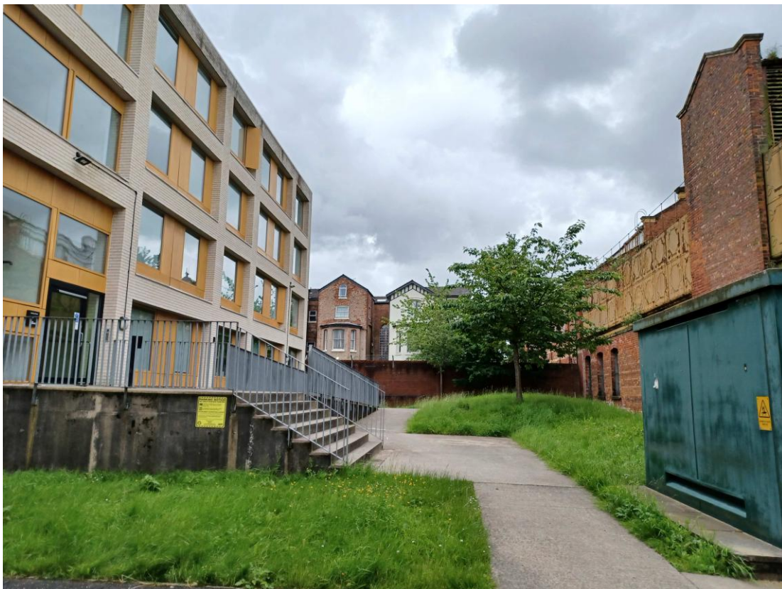
View North towards the rear of 42 and 40 Hathersage Road – Block 1 to the left and Victoria Baths to the right
