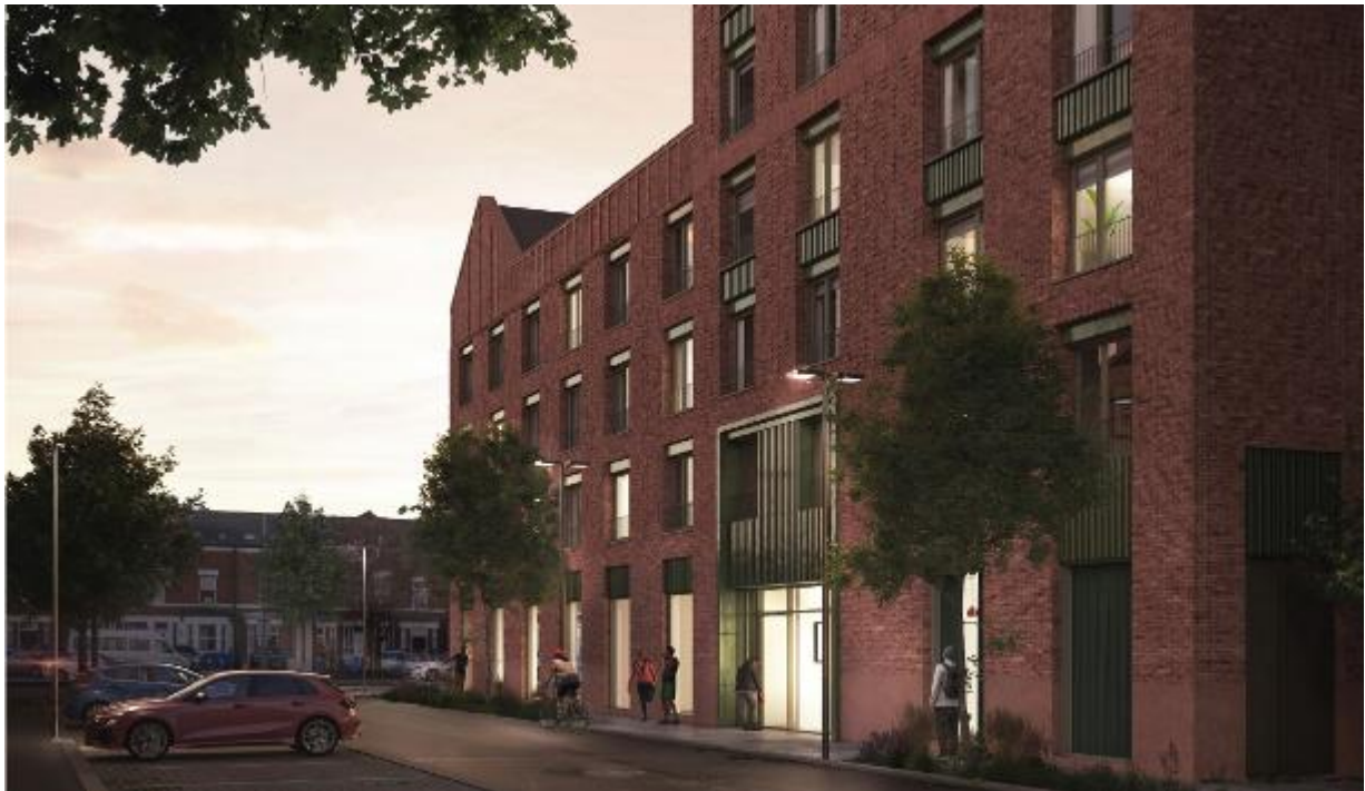
View south along Bax Road towards Hathersage Road with Blocks 5 and 6 to the right
