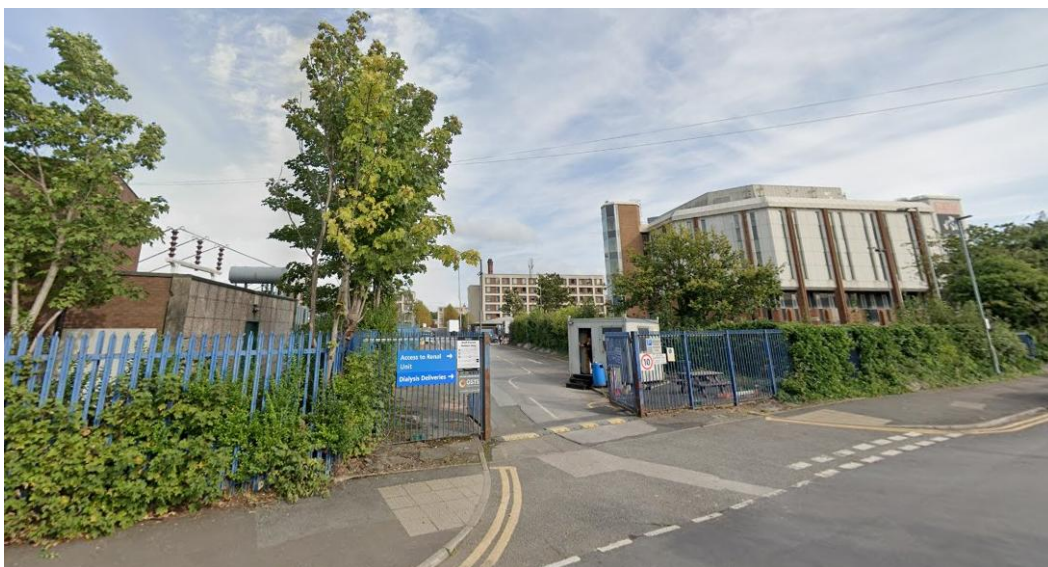
View east towards Block 4 (centre) with the access road from Carmoor Road to the land adjacent the application site and Octagon House (to the right)
