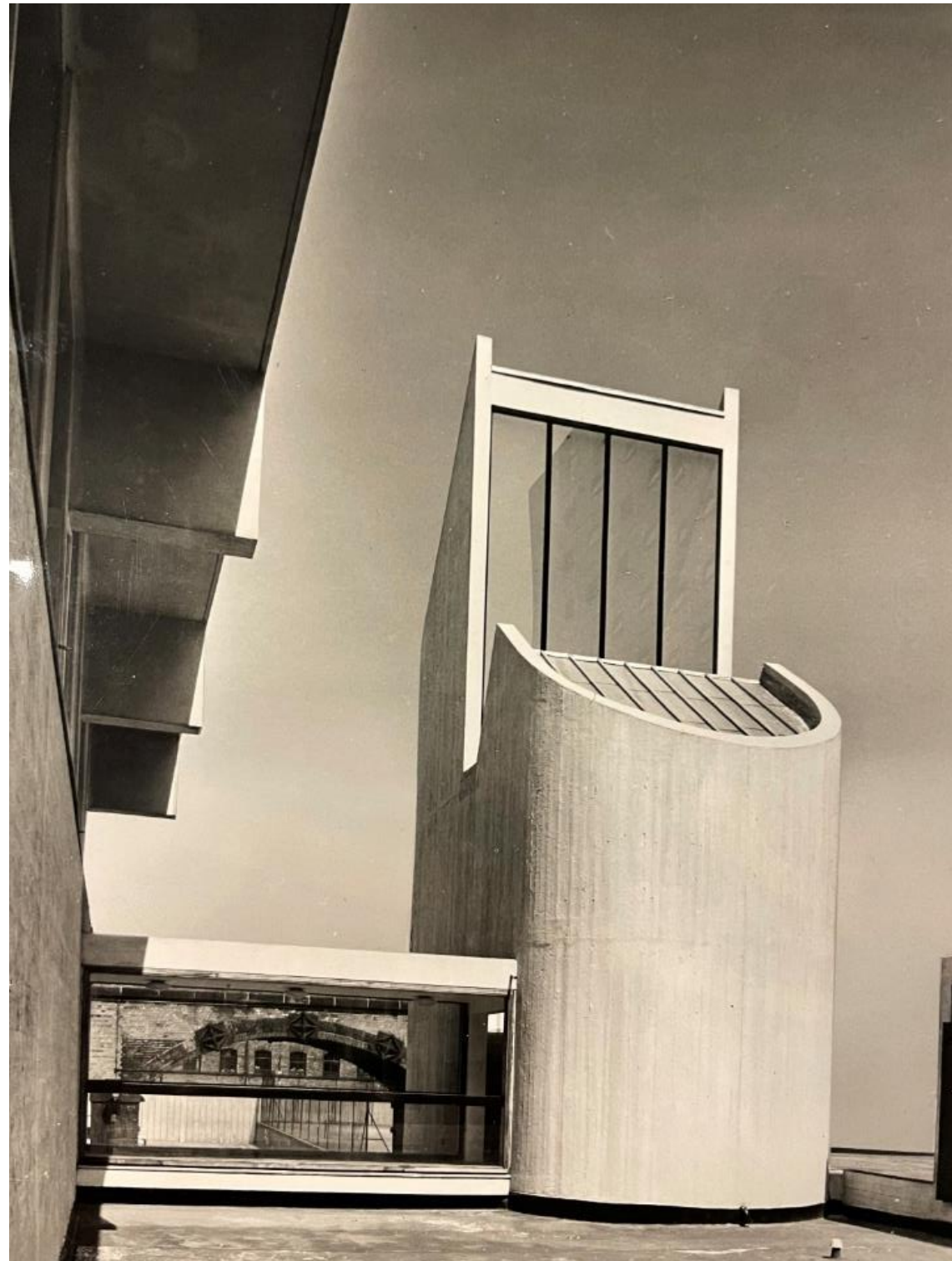
Figure 56: View from the second-floor roof level of the secondary stair tower and the glazed link with the large meeting hall 'The Architects and Builders News', July 1966 (source: Cruickshank & Seward Archives)
