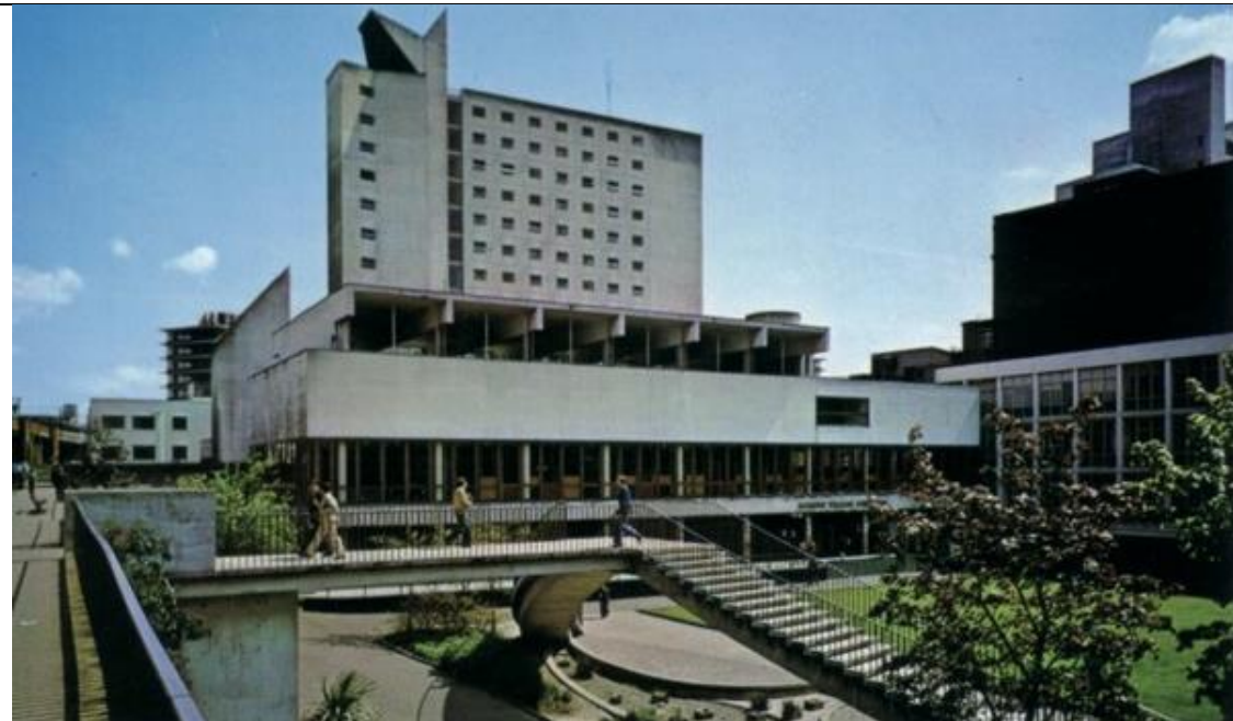
Figure 81: 1970s postcard showing that the original pool beneath the stairs had been infilled by this date, with large stones placed on top.
