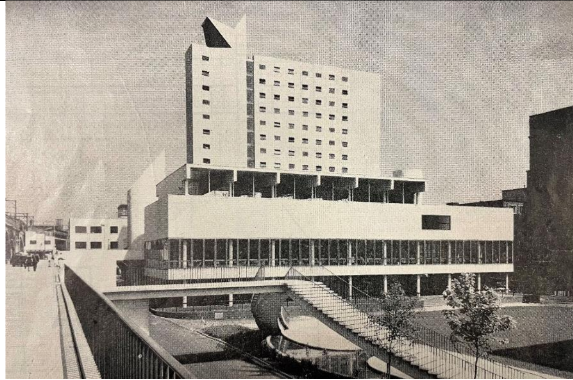
Figure 80: A view looking east towards the Barnes Wallis Building from Altrincham Street in 1966, showing the clear level difference and how the staircase forms an artistic response to both the level difference but also the architecture of the newly completed surrounding college buildings, showing the original reflective pool beneath the stairs. (Source: The Architect and Building News, 27th July 1966)
