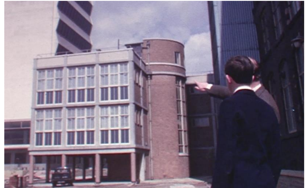
Figure 31: Looking at the west elevation of the Staff House in c.1962, showing the semi-circular stair core, metal-framed windows and open colonnade arrangement. The image illustrates the original, very wide space underneath the covered walkway, which has since been infilled in part by later additions. The mill building can be seen to the far right whilst the Renold Building can be seen to the left. Source: MMU Archive, screenshot from archival video.
