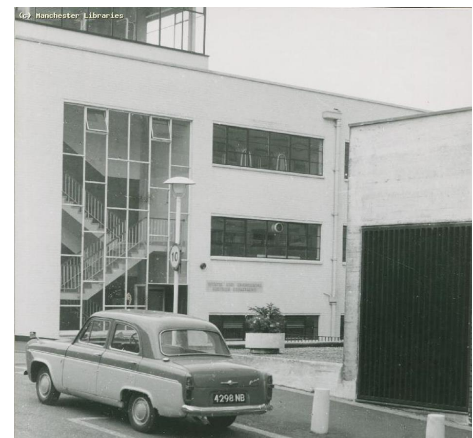
Figure 26: Moffat Building (then known as the estates department), pictured c.1970 from Altrincham Street. West elevation. Note the building is painted white and the elevation is etched with the ‘estates department’. Source: Manchester image archive.
