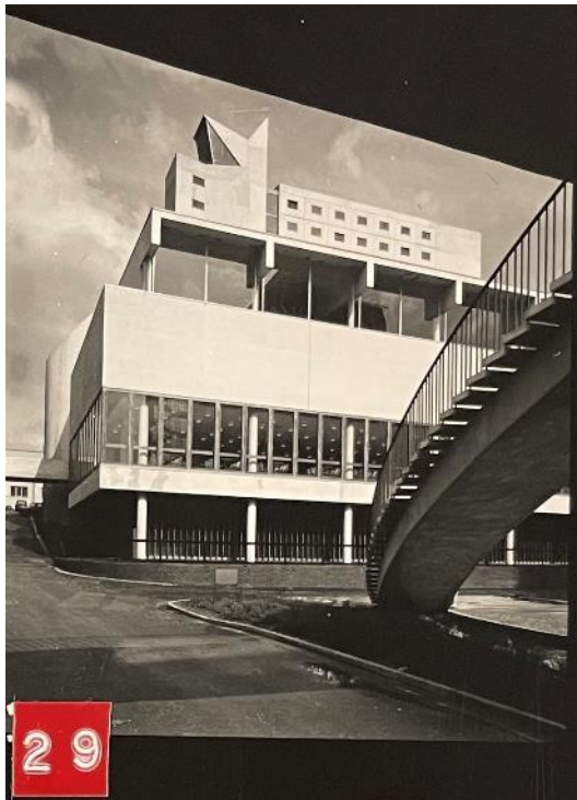
Figure 53: The west elevation as seen from beneath the butterfly stairs in c1966 (source: Cruickshank & Seward Archives)
