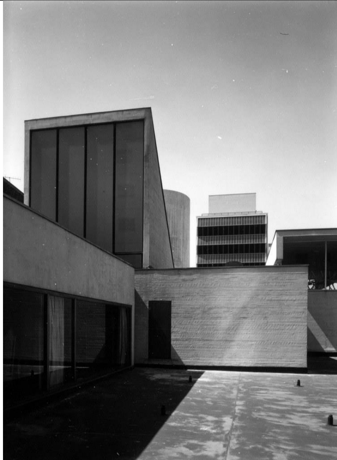
Figure 51: The flat roof area located between the main meeting hall and the full-height council chamber windows (left), to the rear can be seen the large, glazed window that marks the top of the main staircase (source: Cruickshank & Seward Archives).
