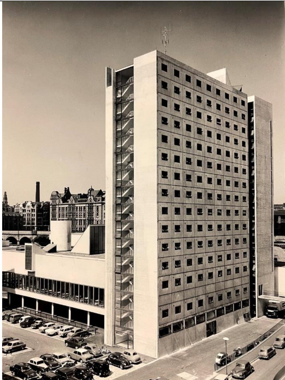
Figure 57: Looking down towards the south (left) and east (right) aspects of the building in c1966, illustrating the interesting architectural shapes used on the flat roof area to the centre of the composition (source: Cruickshank & Seward Archives)
