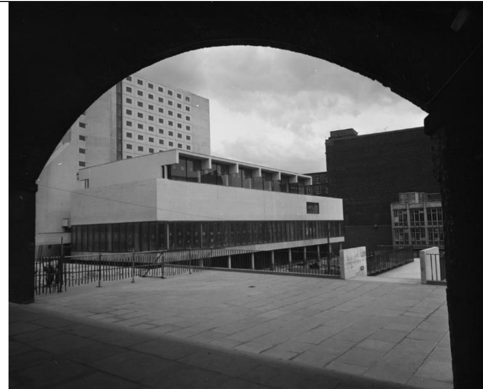
Figure 78: Looking south-east from a railway viaduct arch on Altrincham Street towards the Barnes Wallis Building, showing the approach to the top of the butterfly stair in 1965.
