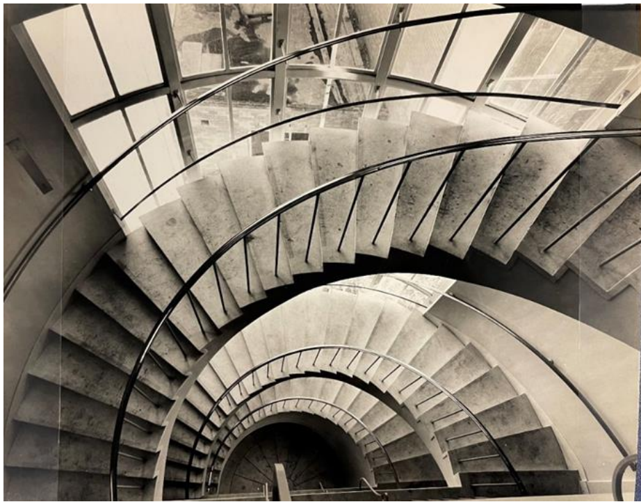
Figure 35: c1960/1 Looking down into the main, semi-circular, cantilevered staircase from the third-floor level, which at this time lead only onto the flat roof. Reinforced concrete and buff terrazzo stairs with brass handrail and semi-circular detailing to the ground floor terrazzo, and full height, metal-framed windows. Source: MMU Archive.
