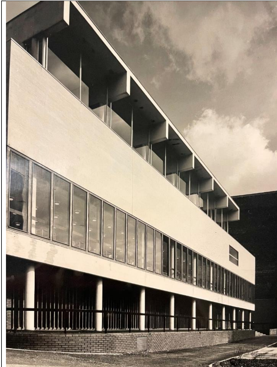
Figure 58: The west elevation as seen in c1966 (source: Cruickshank & Seward Archives)
