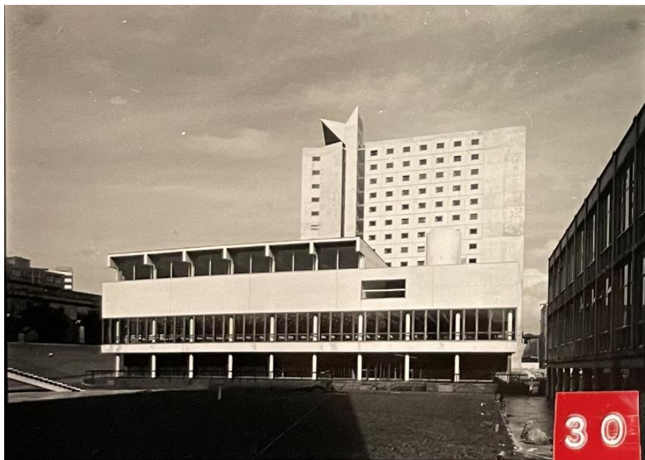
Figure 55: The west elevation as seen the western side of the bowling green in c1966 (source: Cruickshank & Seward Archives)
