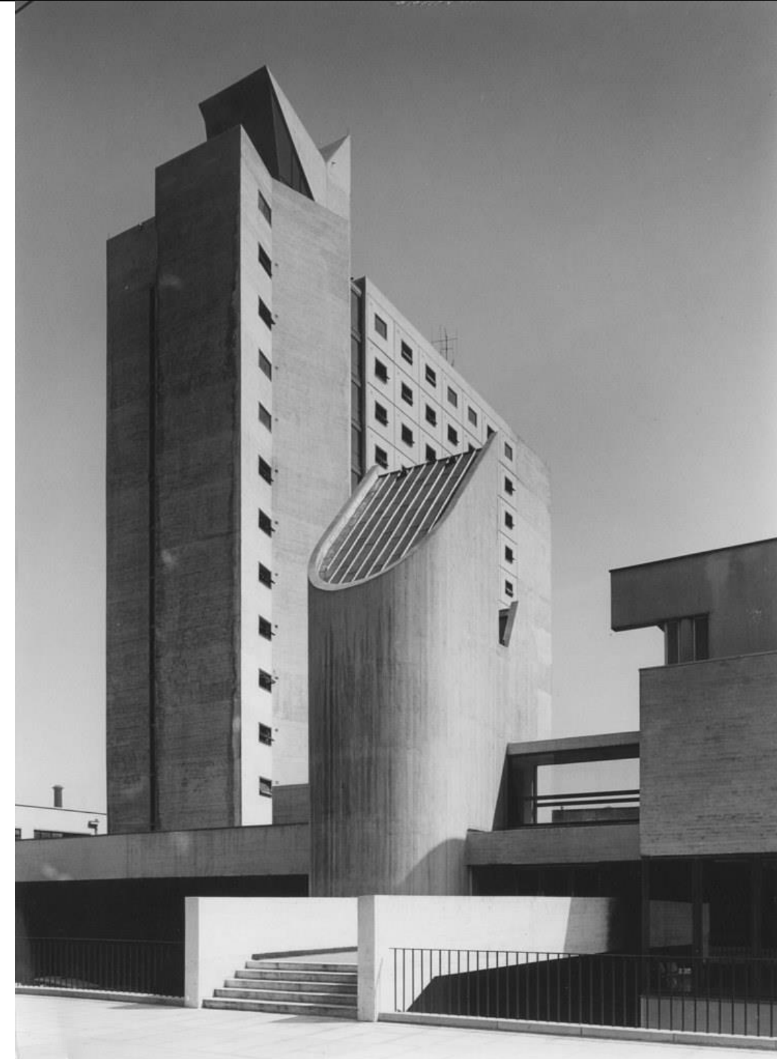
Figure 52: Looking towards the north elevation from Altrincham Street, showing the first-floor bridged entrance (centre) and windows of the former cafeteria (right). The curved concrete structure forms an internal staircase (source: Cruickshank & Seward Archives)
