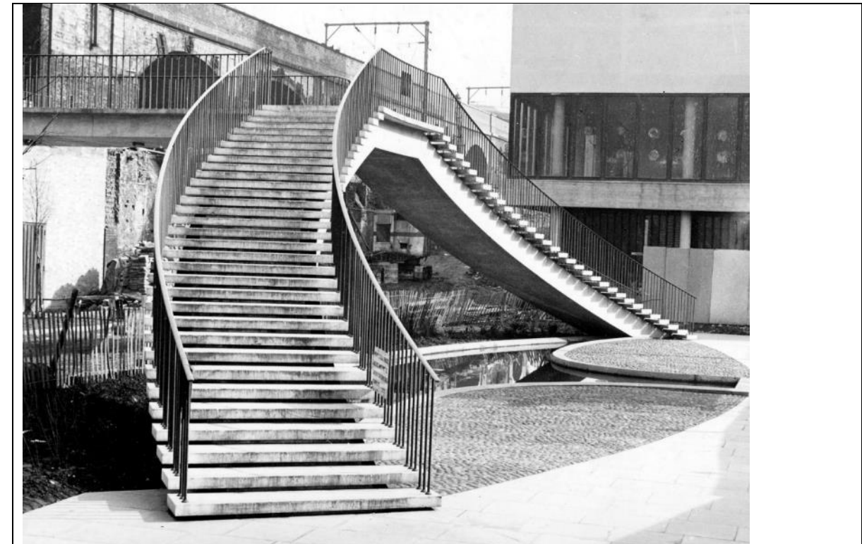
Figure 76: Concrete butterfly stair, pictured in 1965. The sweeping form of the stair and balustrade is represented well in the image. The ornamental reflective pool and cobbles described within the 1963 article above are also visible. The Barnes Wallis building is seen under construction to the right.
