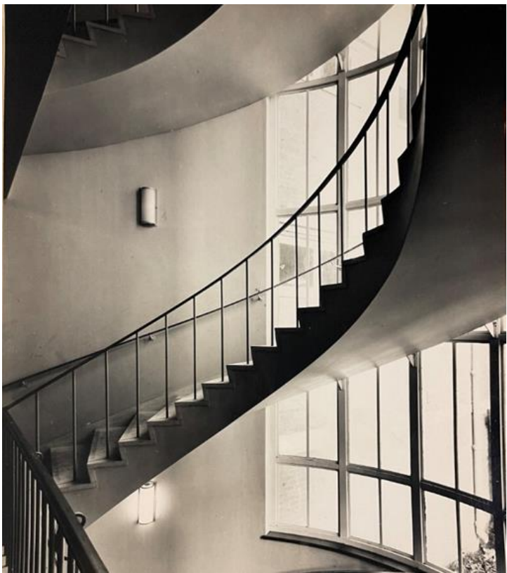
Figure 35: c1960/1 Looking down into the main, semi-circular, cantilevered staircase from the third-floor level, which at this time lead only onto the flat roof. Reinforced concrete and buff terrazzo stairs with brass handrail and semi-circular detailing to the ground floor terrazzo, and full height, metal-framed windows. Source: MMU Archive.
