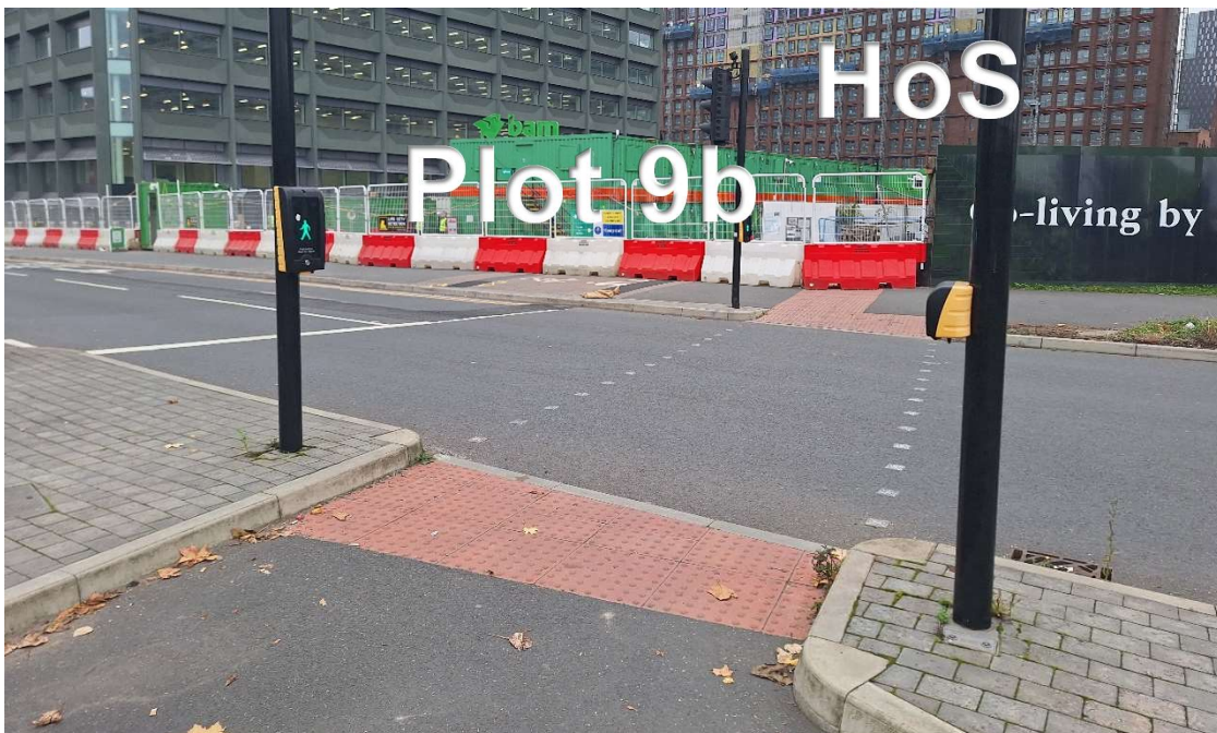
Figure 8 Medlock Street Signal Toucan Crossing with Tactiles, Audible signal and Tactile Cone
