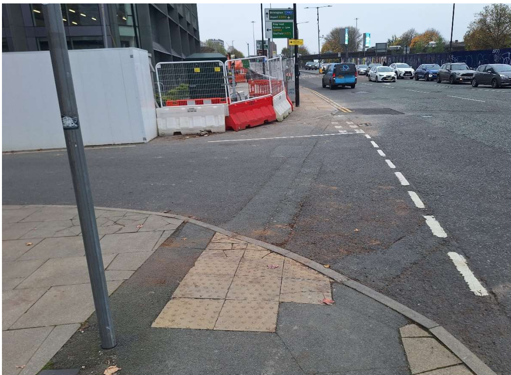
Figure 6 Pedestrian Crossing of River Street (E)
