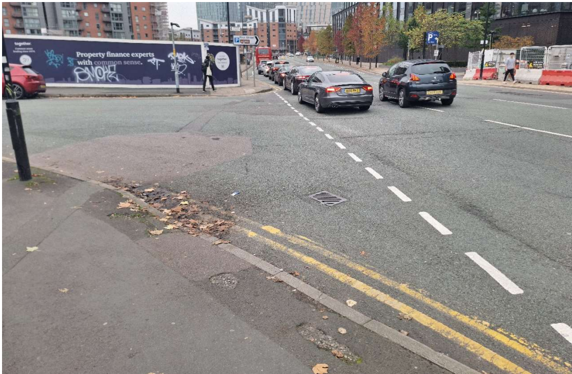
Figure 7 Pedestrian Crossing of River Street (W)
