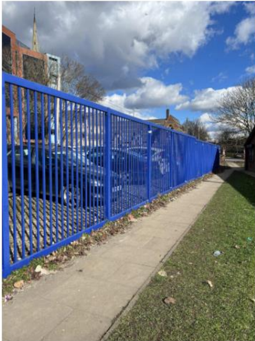
1 - View of existing fence looking down footpath towards Chichester Road S.
