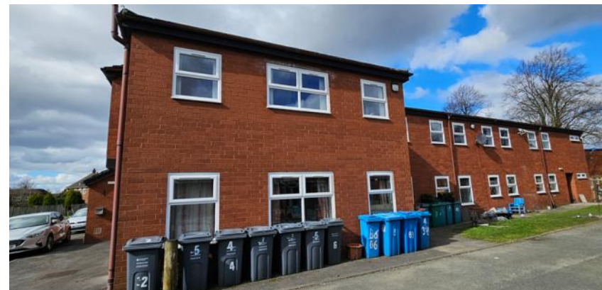
Below - View facing eastern side of 1 Cornish Close
