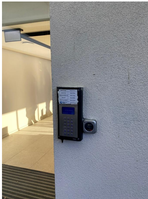
Photograph 6 – Access Control to Main Entrance
