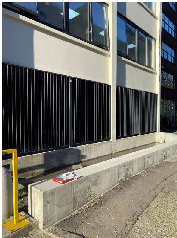
Photograph 2 – Full height railings (Major St)
