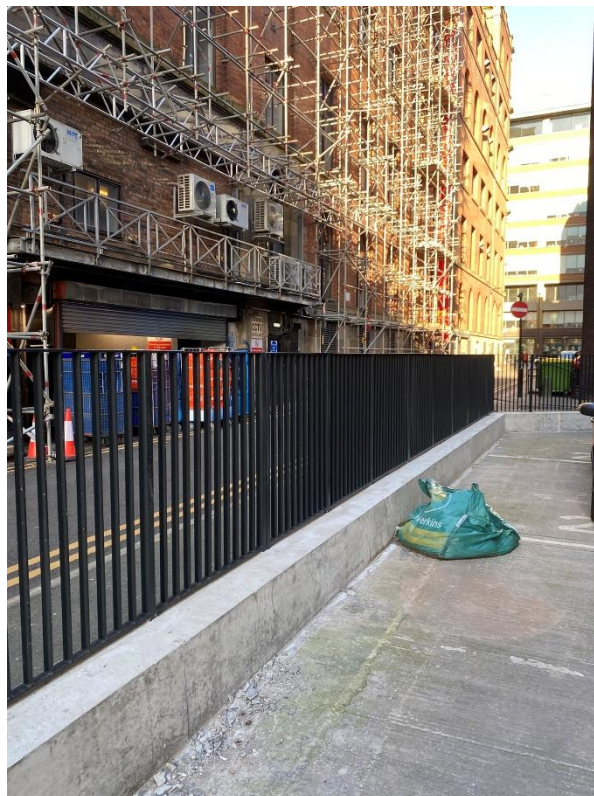
Photograph 4 – New railings (Siver & Gold St)
