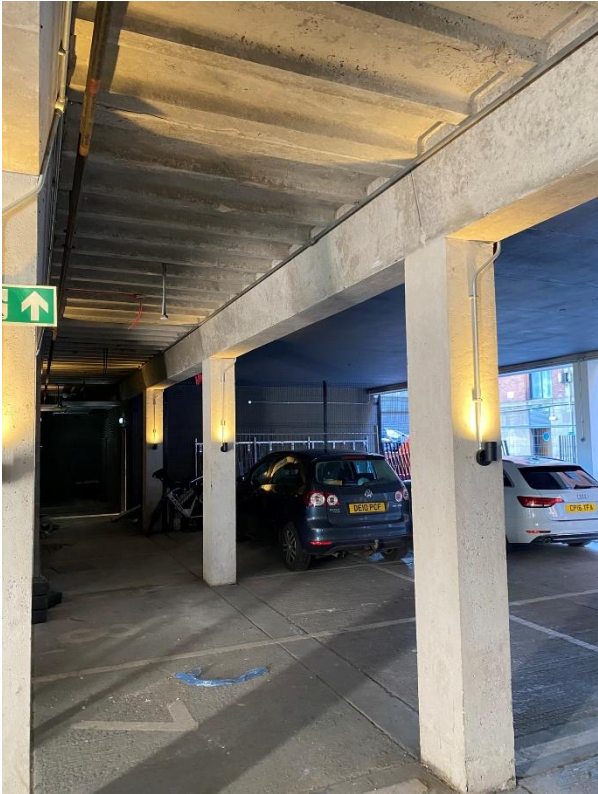
Photograph 9 – New lighting to car park to improve illumination
