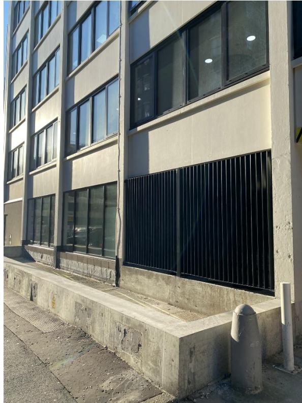
Photograph 3 – Full height railings (Major St)
