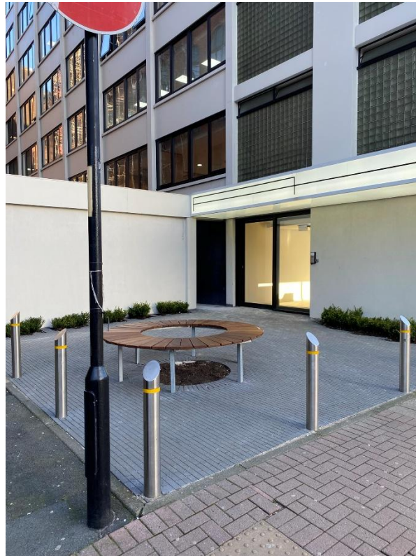
Photograph 5 – Anti-ram bollards
