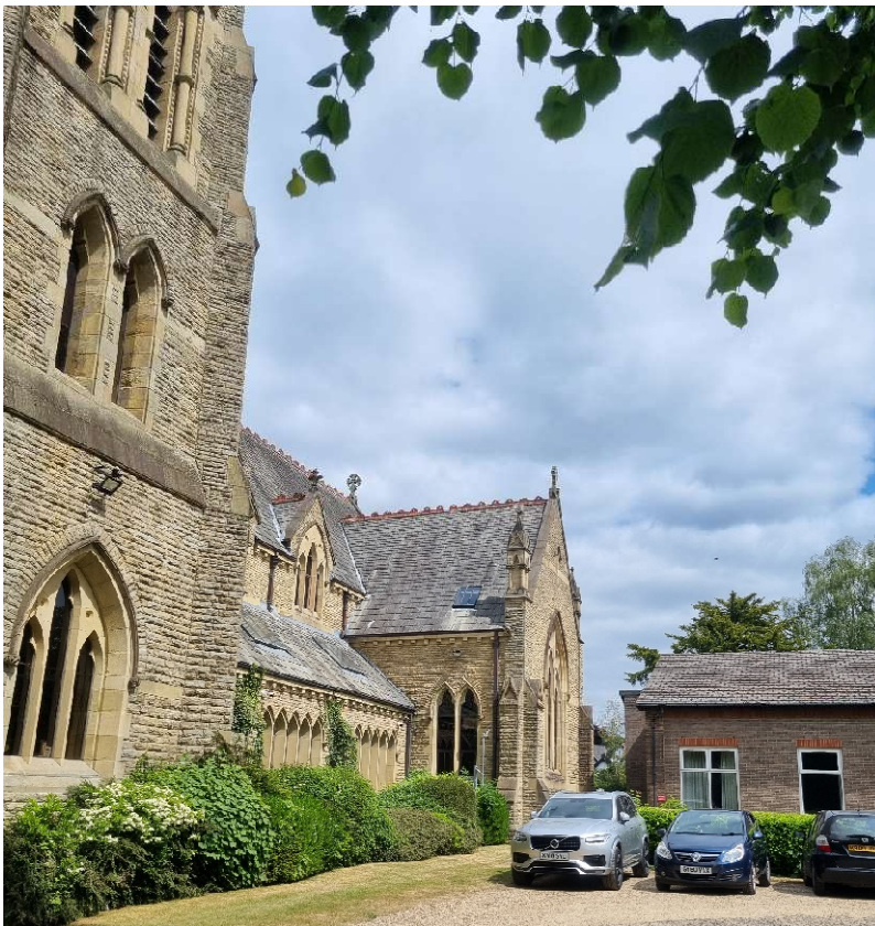
Fig 4 View : Relationship between the two buildings
