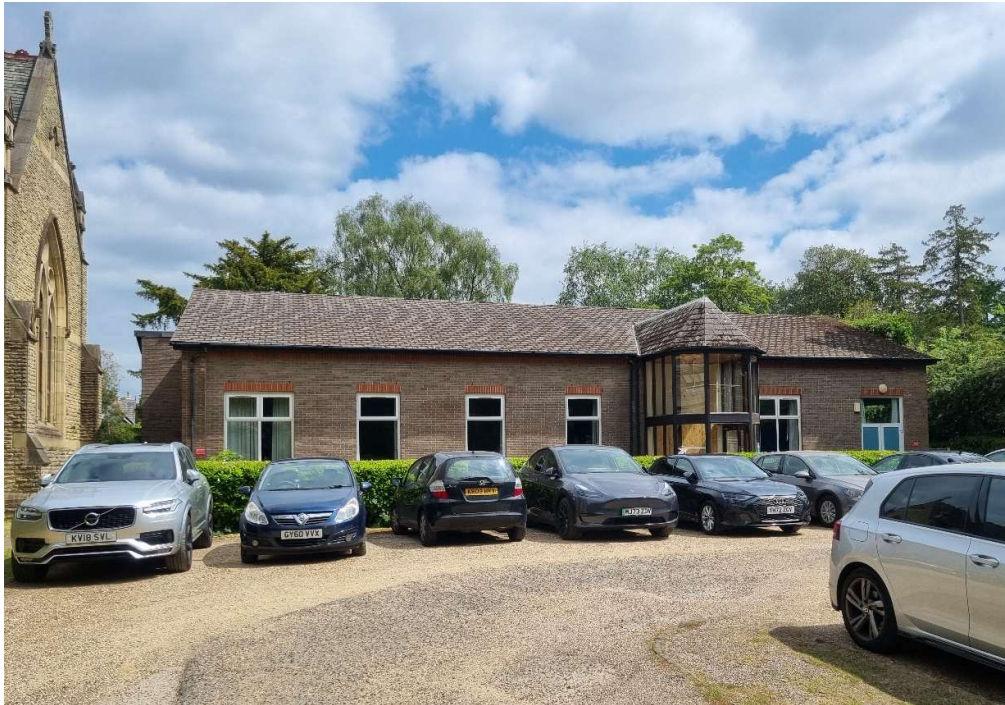
Fig 5 View to Former Methodist Church (West Elevation)
