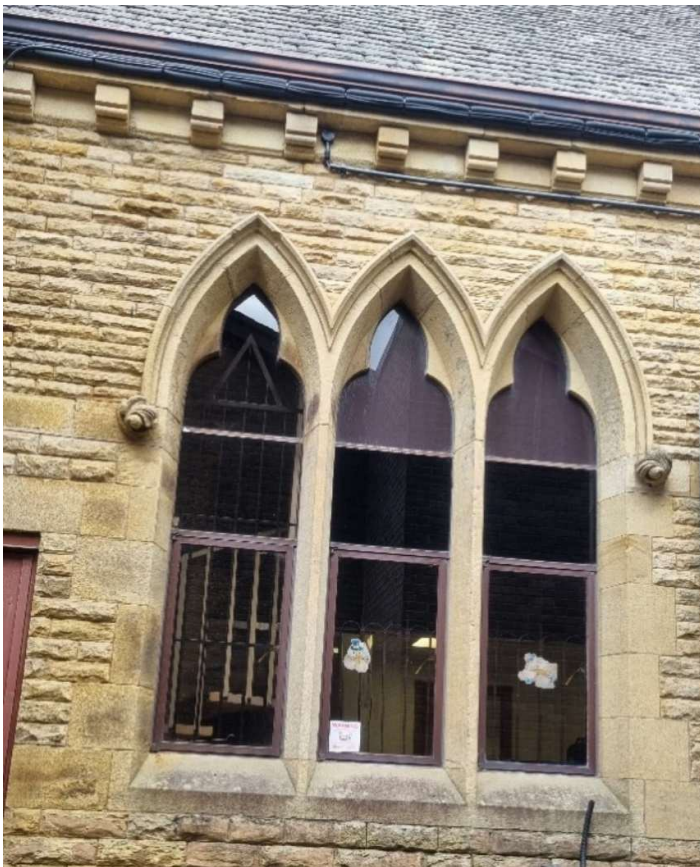
Fig 9 Photograph showing elevation and window affected by proposed link
