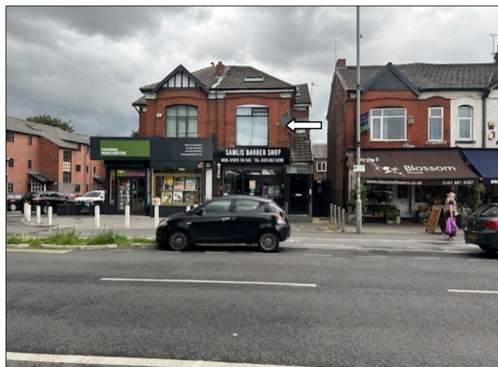
View of application property frontage
