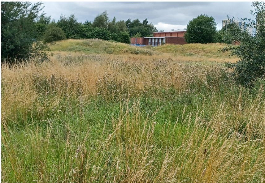
View looking westwards from Hinchley Road to the Manchester Creative and Media Academy buildings
