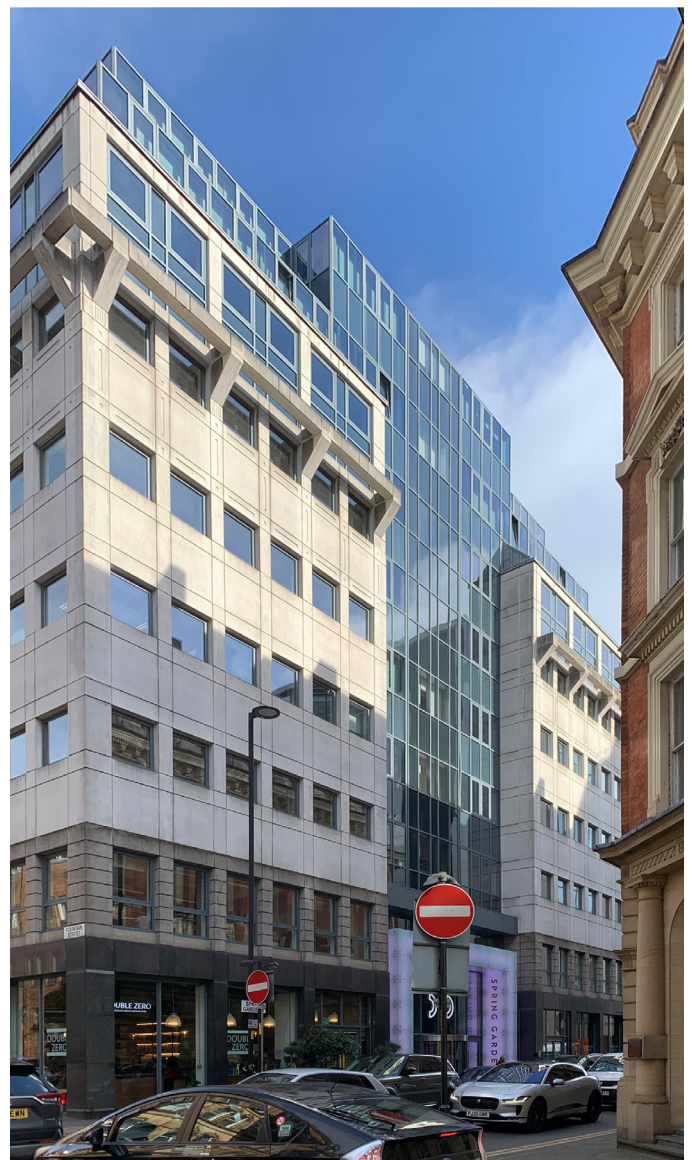
Existing Building - View from Fountain Street
