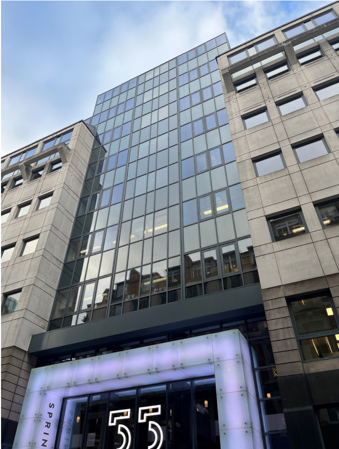
Existing Curtain Walling Facade
