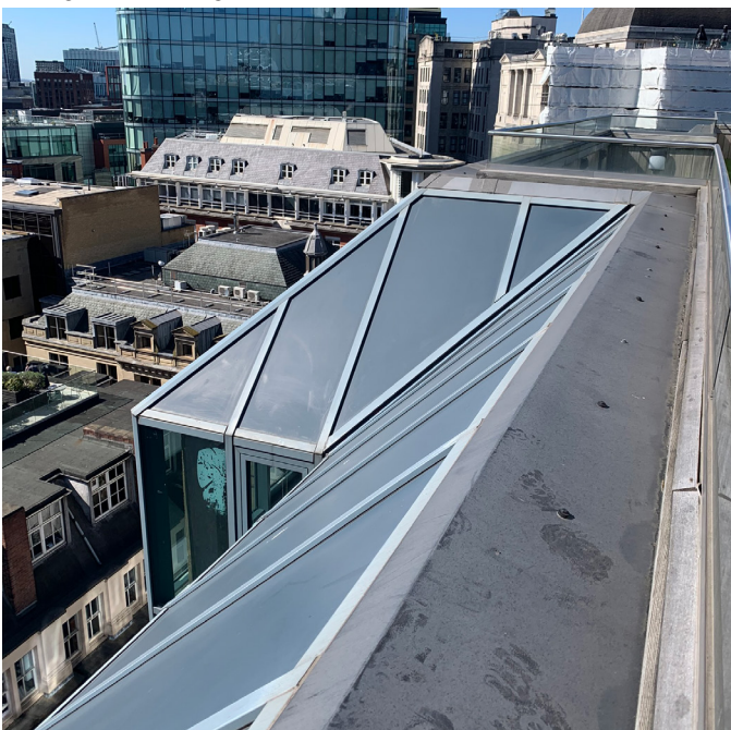
Spandrel Panels at Level 9
