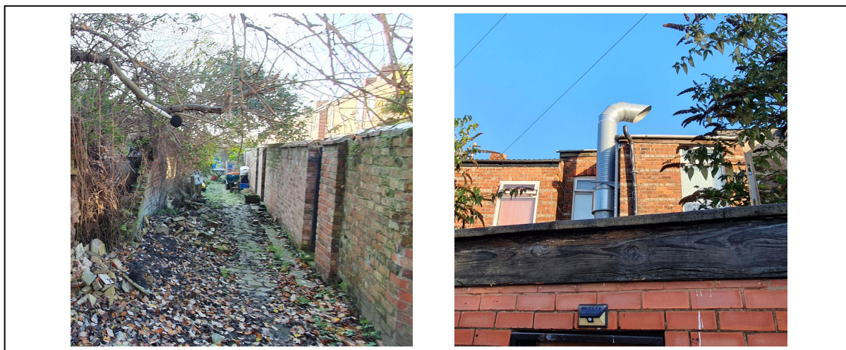
Figure 3: Site Location Measurement Pictures
