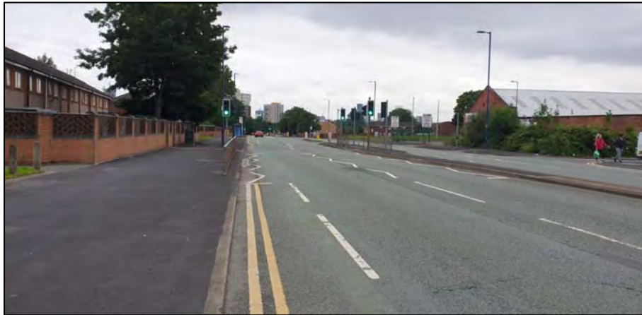
Image 2.4 Signalised Pedestrian Crossing on Oldham Road
