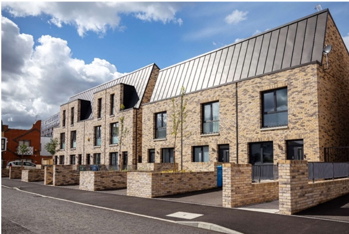
Housing at Mulino Walk, forming part of the Downley Drive development in New Islington, Manchester
