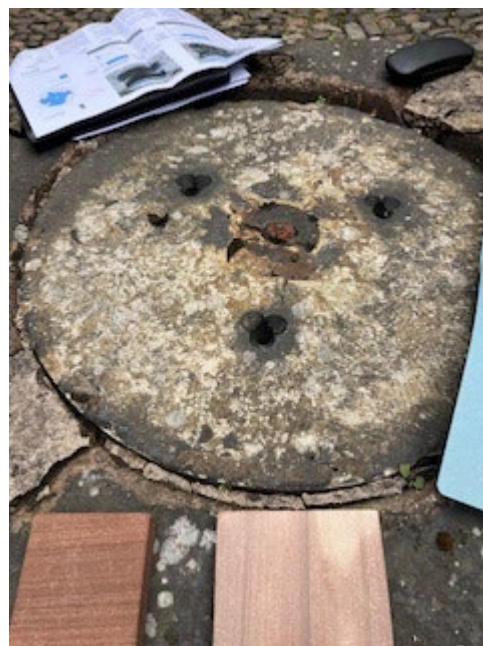
Fox's Court Well central stone to retain.
