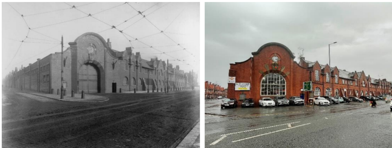
Figure 1: Views of the south elevation of the former tram shed (now bus depot) from the south west on Queens Road; 1902 (left) and 2025 present day (right).
